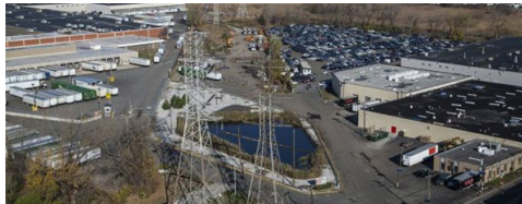
PSE&G's Kingsland-Hudson reliability project in Kearny, N.J. | Kiewit
