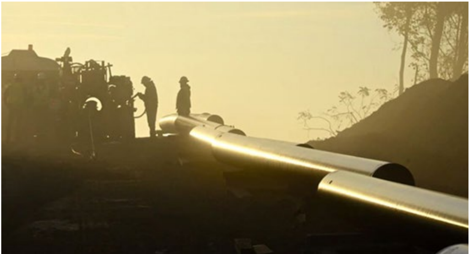
Natural gas pipeline construction | Williams
