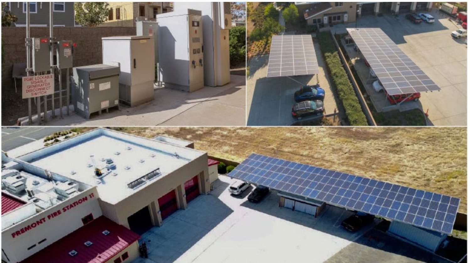
The city of Fremont, Calif., employs solar and battery storage to power critical facilities such as fire stations. | City of Fremont
