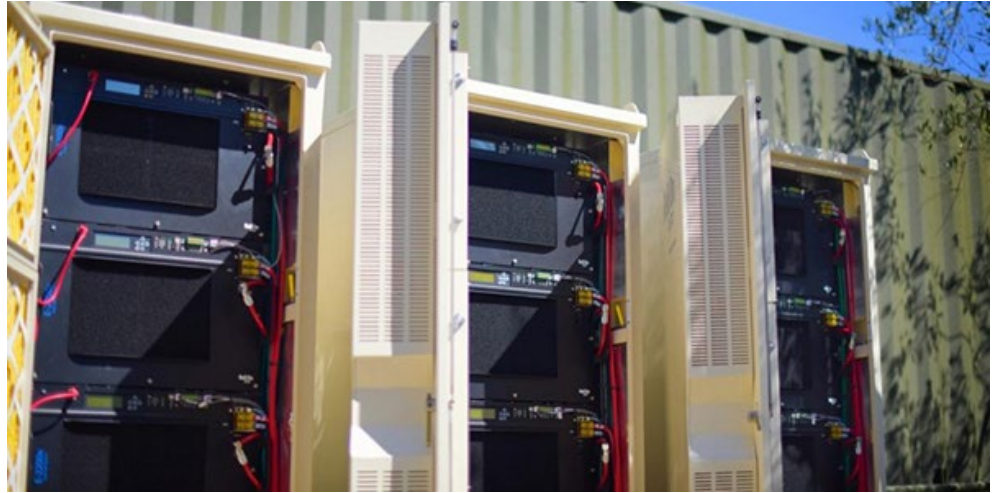
Stone Edge Farm in Sonoma County, Calif., uses an electrolyzer and hydrogen fuel cells to store solar energy for use during the winter rainy season. | Stone Edge Farm
