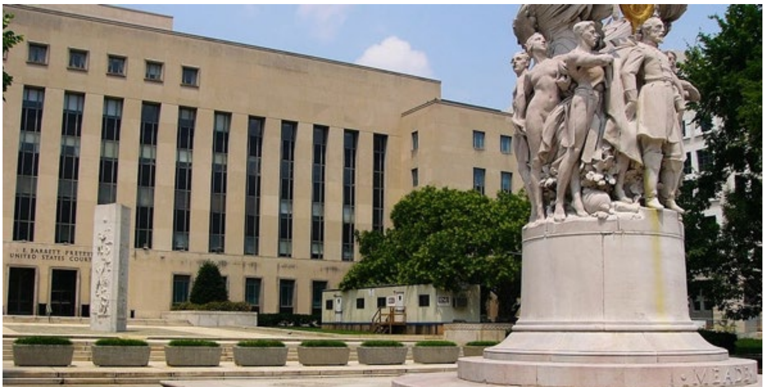
E. Barrett Prettyman Federal Courthouse, home of the D.C. Circuit Court of Appeals | HSU Builders
