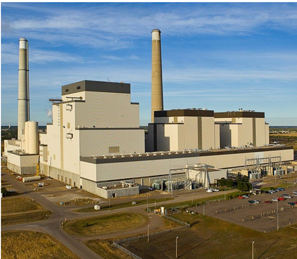
Sherco Generating Station | Xcel Energy
