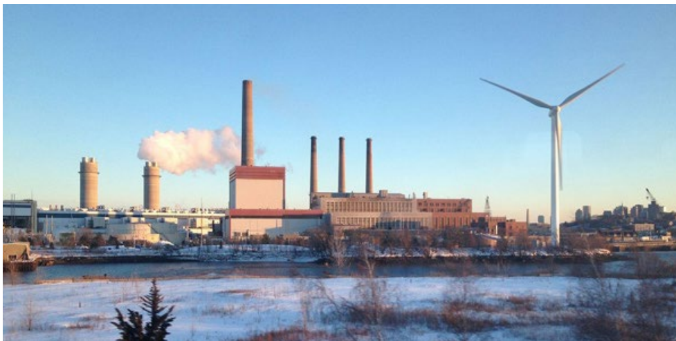
Exelon's Mystic Generating Station, on the Mystic River in Everett, Mass. A wind turbine owned by the local water authority to power a pumping station is on the right.
