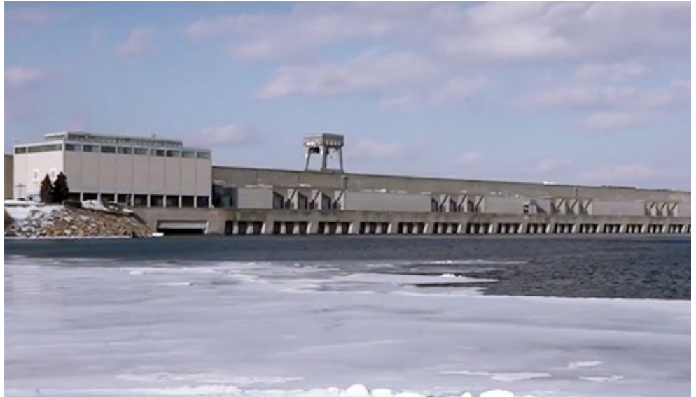
St. Lawrence-Franklin D. Roosevelt Power Project on the St. Lawrence River | NYPA
