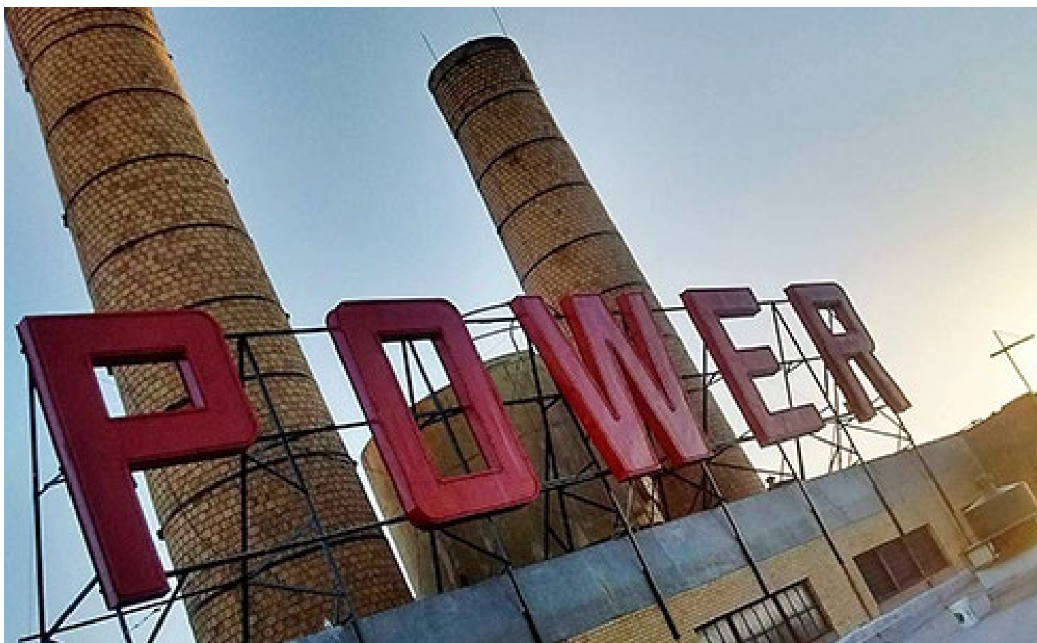
EPE's Rio Grande Plant in Sunland Park, N.M. | El Paso Electric
