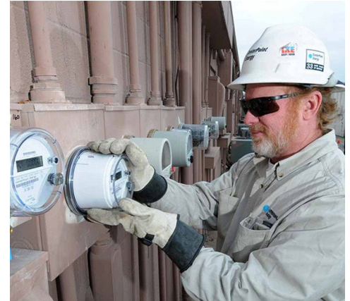
A CenterPoint Energy serviceman checks a gas meter. | CenterPoint Energy
