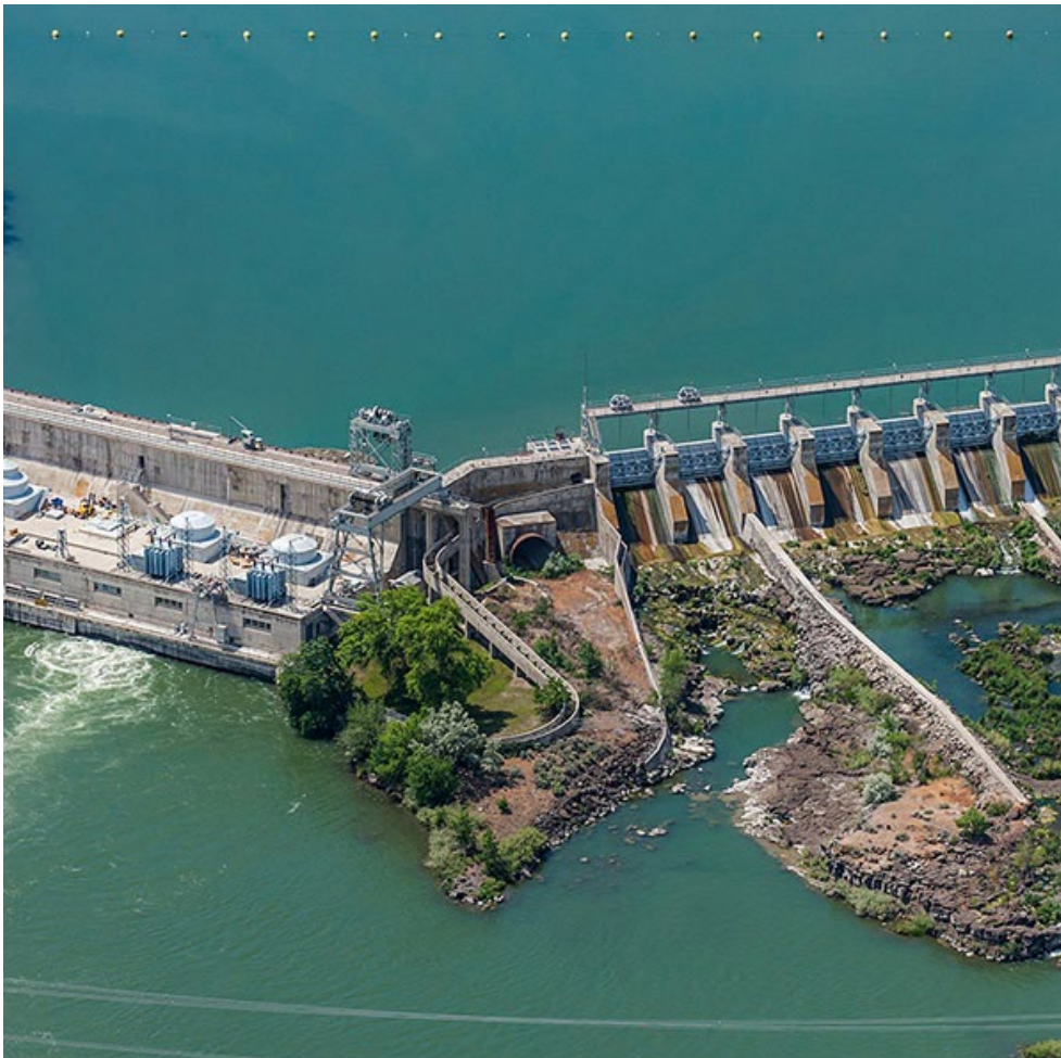
Lower Salmon Dam | Idaho Power
