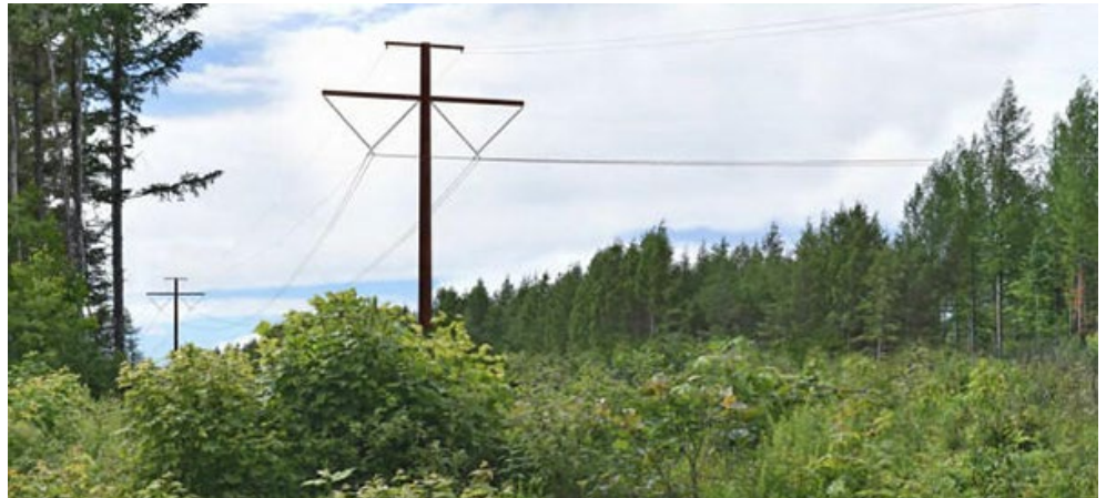
A rendering of what the poles will look like along CMP's 145-mile transmission line | Central Maine Power
