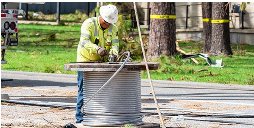
Restoration worker handling new wires | Entergy
