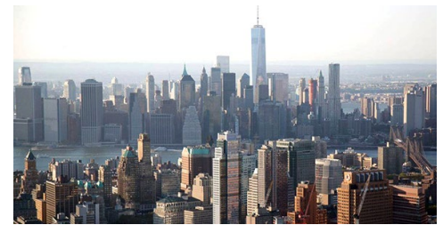
Con Edison won approval from the NYISO BIC of a proposal to increase the exemption from real-time generation penalties for units that supply steam to New York City. | Con Edison
