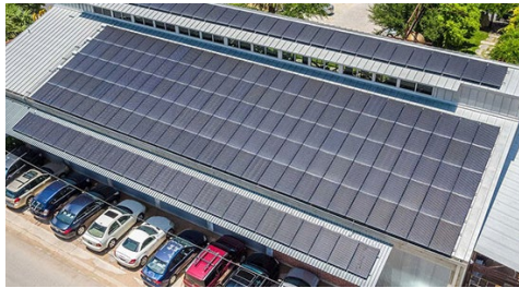
Freedom Solar Power's 50-kW solar array on an architects' office building in San Antonio | Freedom Solar Power
