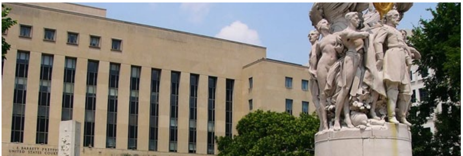
E. Barrett Prettyman Federal Courthouse, home of the D.C. Circuit Court of Appeals | HSU Builders
