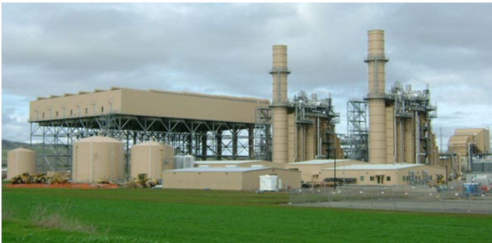
PG&E's natural-gas fired Colusa Generating Station | PG&E
