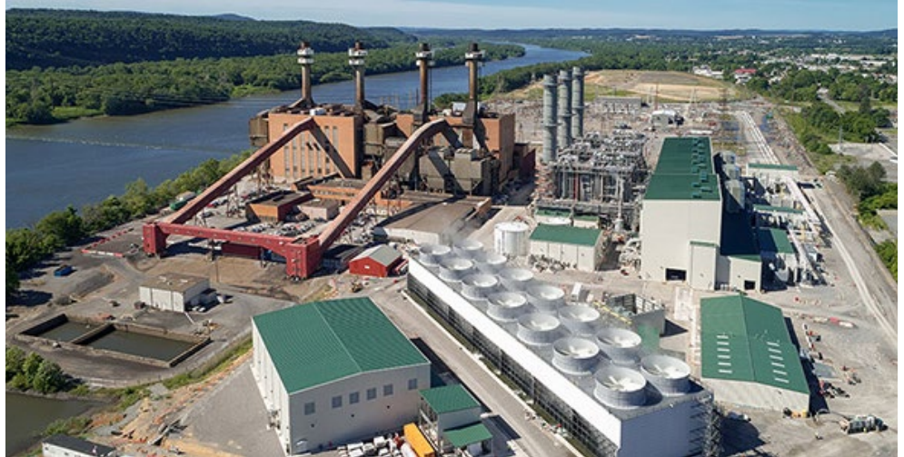
Panda Hummel Station, a 1,096.5-MW combined cycle plant on the Susquehanna River near Sunbury, Pa. | Bechtel Corp.
