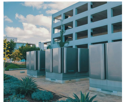
Bloom Box energy servers using solid oxide fuel cells | Bloom Energy
