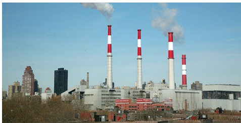
Ravenswood Generating Station, a 2,480-MW fossil fuel plant in New York City
