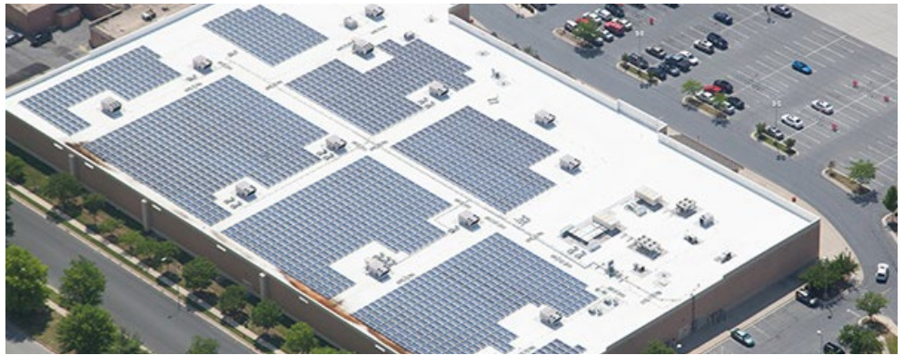
Solar panels cover the roof of a Target store in Middle River, Md. | Chesapeake Bay Program
