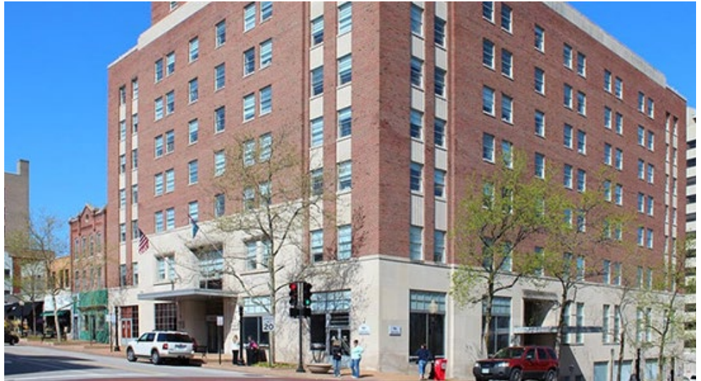
The Missouri PSC office building in Jefferson City, Mo. | Richard A. Howerton Properties & Development
