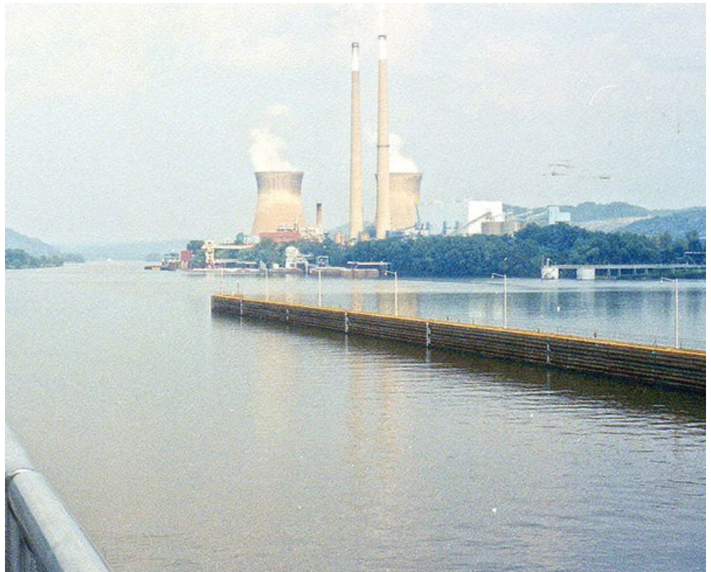
The coal-fired Pleasants Power Station in West Virginia
