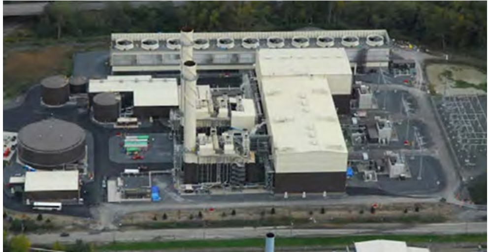
The 635-MW Empire Generating facility in Rensselaer, NY | Empire
