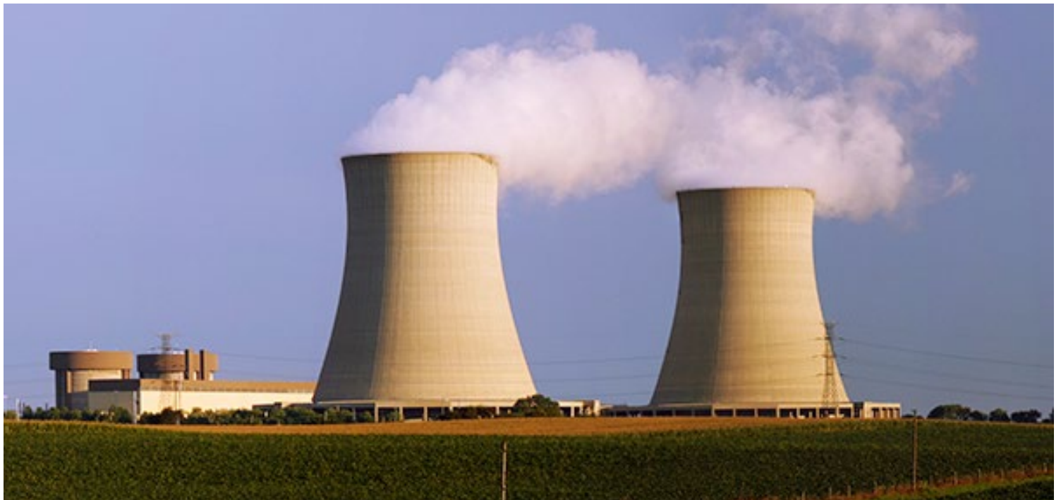
Exelon’s Byron Generating Station’s two nuclear reactors in Illinois produce more than 2,300 MW.
