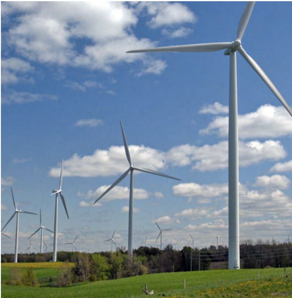
The Marble River Wind Farm along the Canadian border in Clinton County, N.Y. | NYSEERDA
