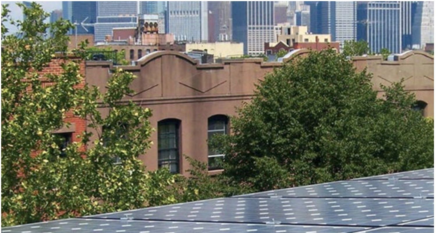
Rooftop solar panels in Brooklyn | NYSERDA
