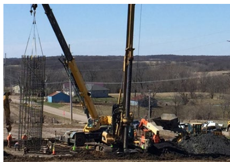
Ameren line construction | Plocher Construction
