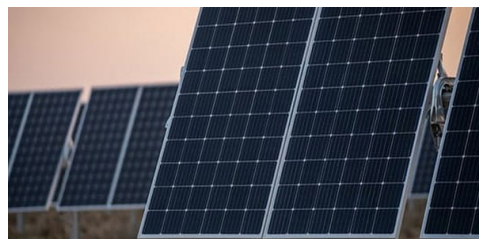
Solar resources, like the Permian Solar Center, account for much of ERCOT's recent additional capacity. | Ørsted
