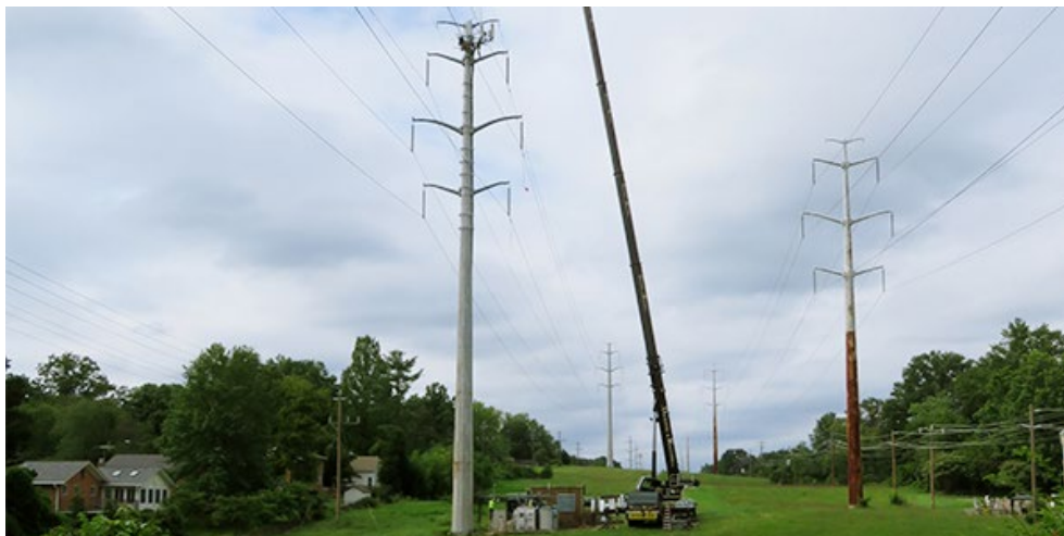
Crane lifts workers to top of transmission tower in Potomac, Md. | © RTO Insider
