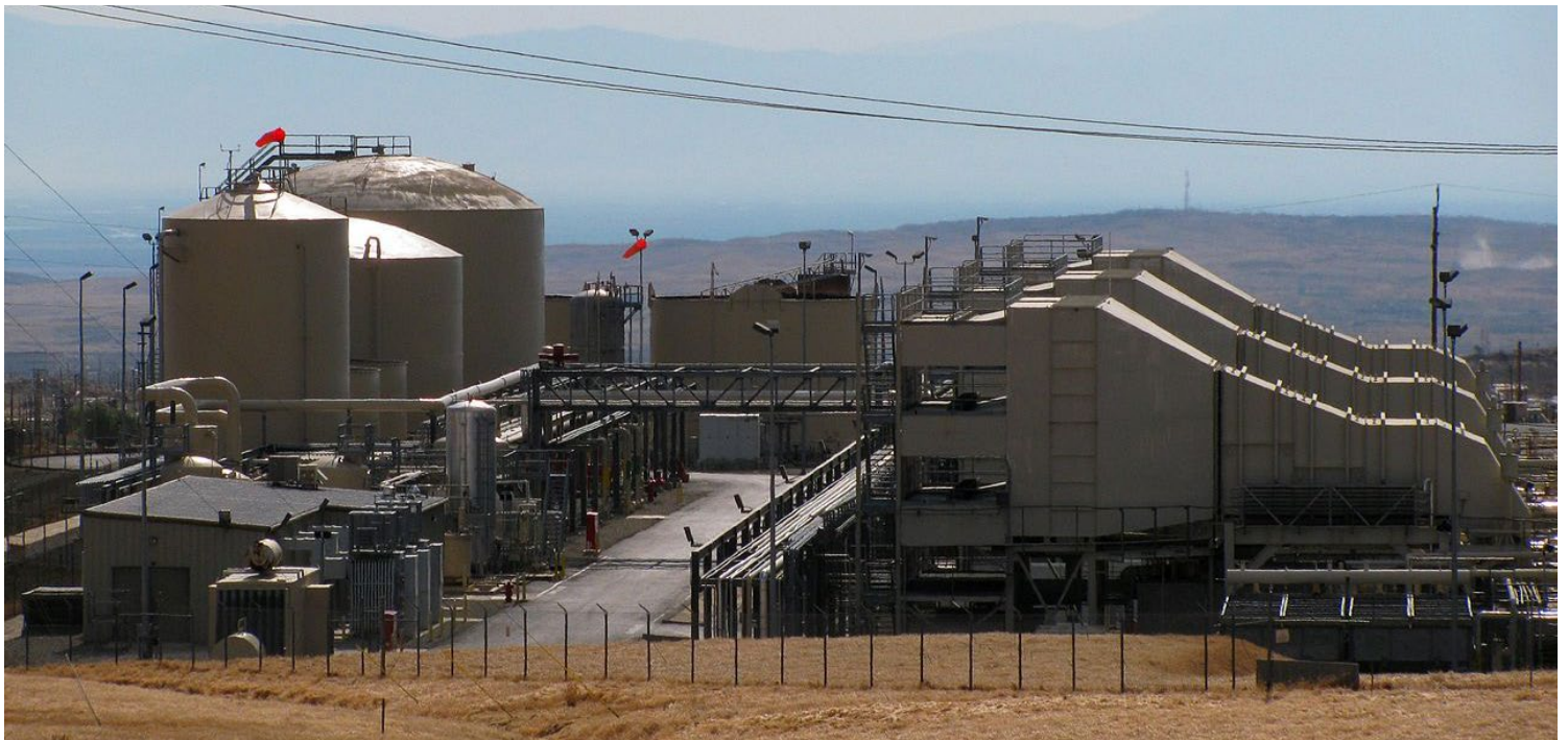
The Midway Sunset Cogeneration plant sits in a Kern County oil field.
