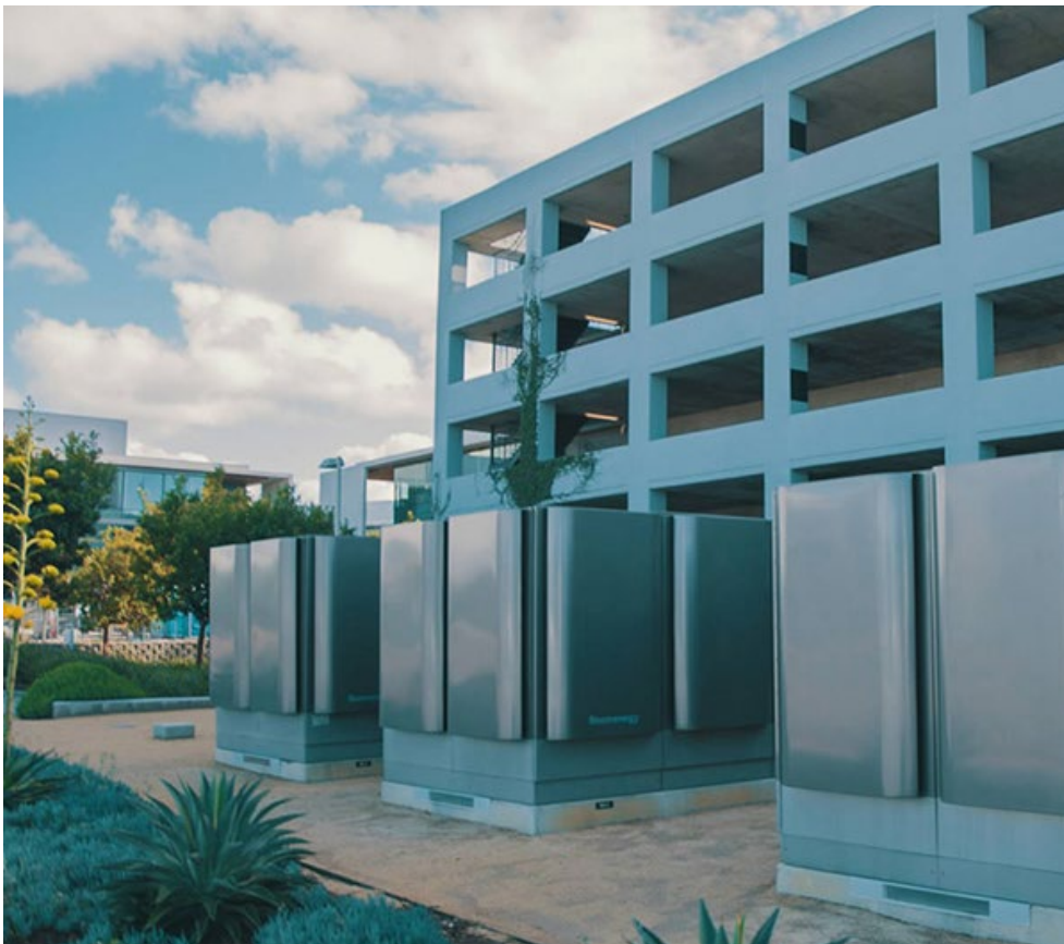
Bloom Box energy servers using solid oxide fuel cells | Bloom Energy
