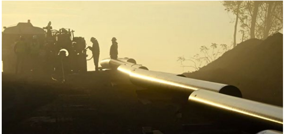
Natural gas pipeline construction | Williams
