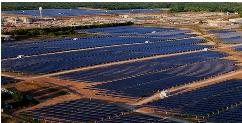
Utility-scale solar facilities are helping pad ERCOT’s reserve margins. | CPS Energy
