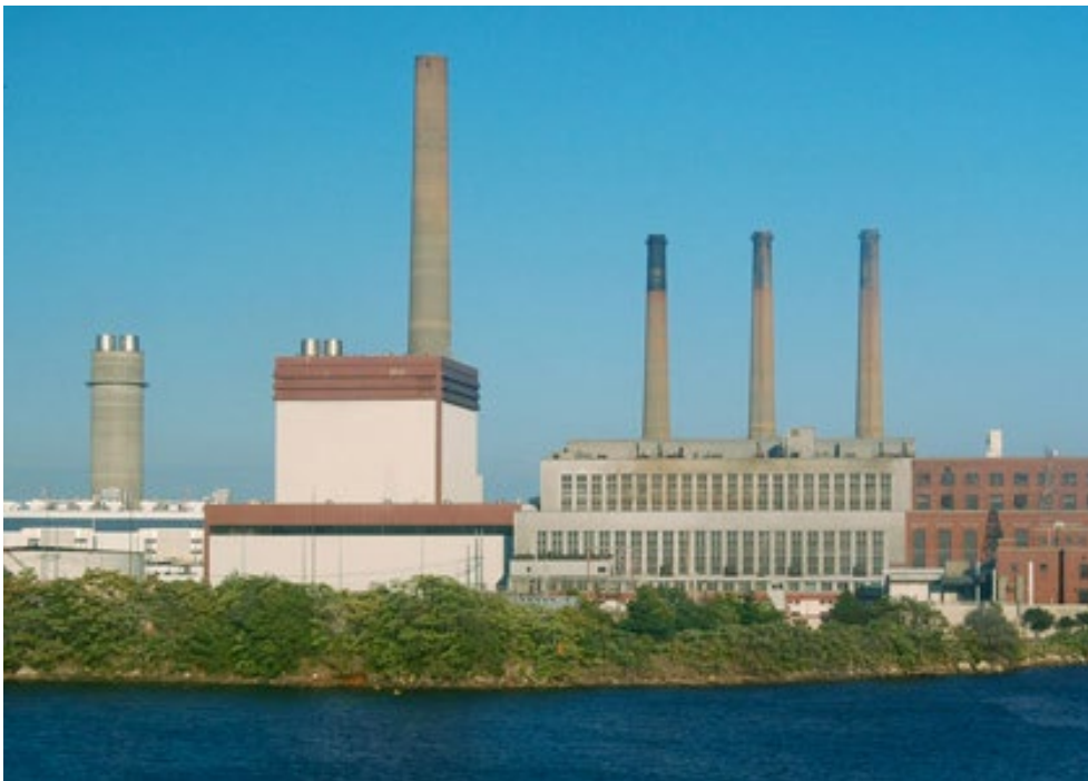
Mystic Generating Station, on the Mystic River in Everett, Mass.
