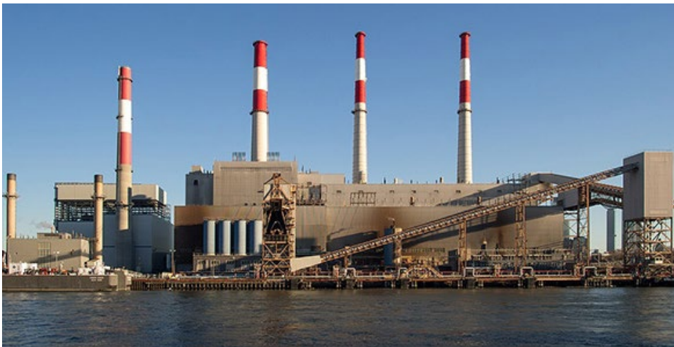
The Ravenswood Generating Station, run by Rise Light & Power, as seen from a neighboring street in Roosevelt Island
