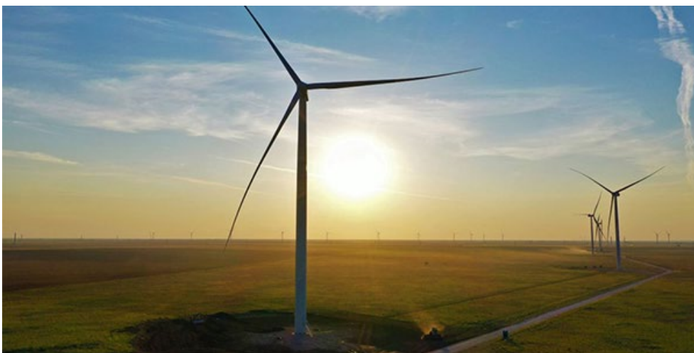
Xcel Energy’s newly energized Sagamore Wind Project in New Mexico has added 522 MW of capacity to SPP’s fuel mix. | Xcel Energy
