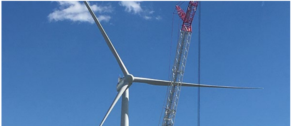
Construction of the Merricourt Wind Energy Center in 2020 | Otter Tail Power
