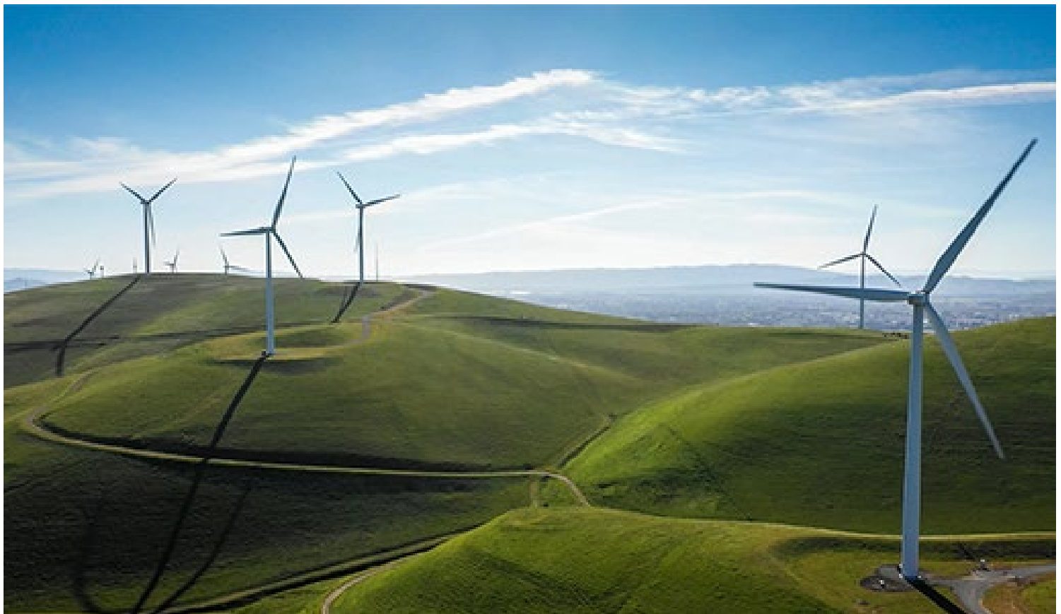
CCAs are banding together to buy renewables and storage. | Silicon Valley Clean Energy
