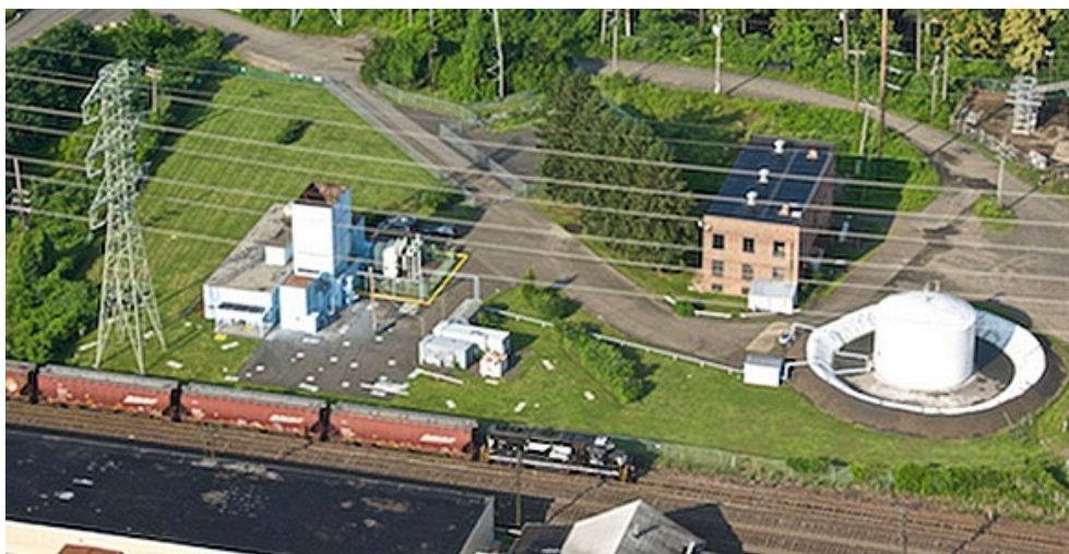
Alliance's 40-MW Hillburn plant in Hillburn, N.Y. | Alliance Energy Group
