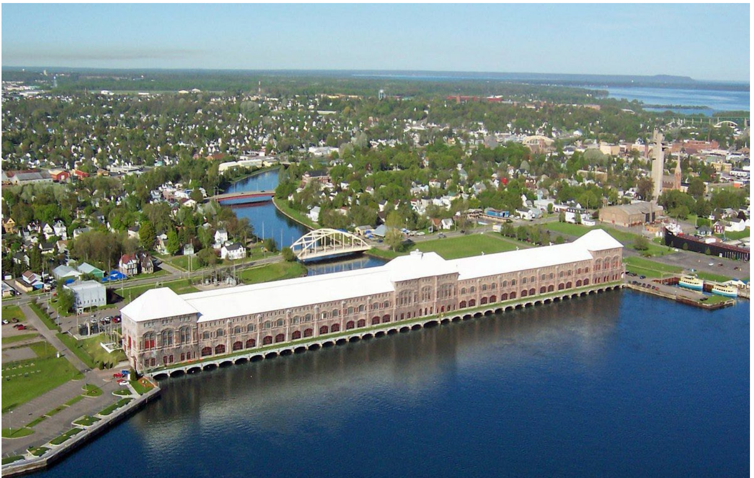
Cloverland's hydroelectric plant in Northern Michigan | Cloverland Electric Cooperative
