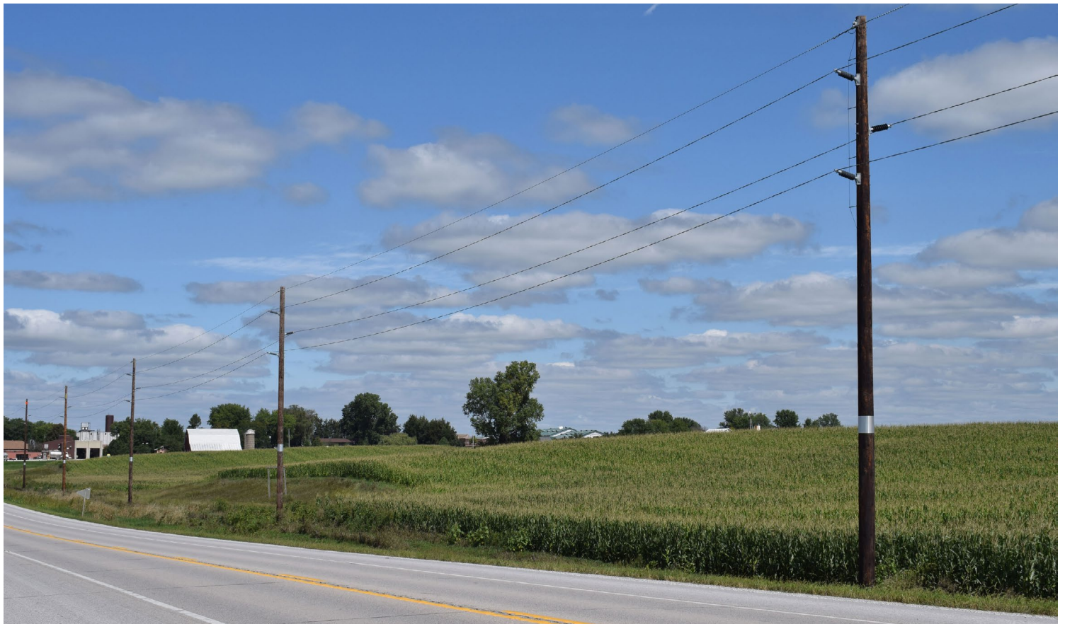
ITC Midwest has been upgrading transmission in Iowa. | ITC
