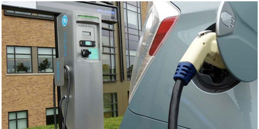
NYSERDA EV chargers: An employee’s vehicle charging at a GE facility in Schenectady, New York | NYSERDA
