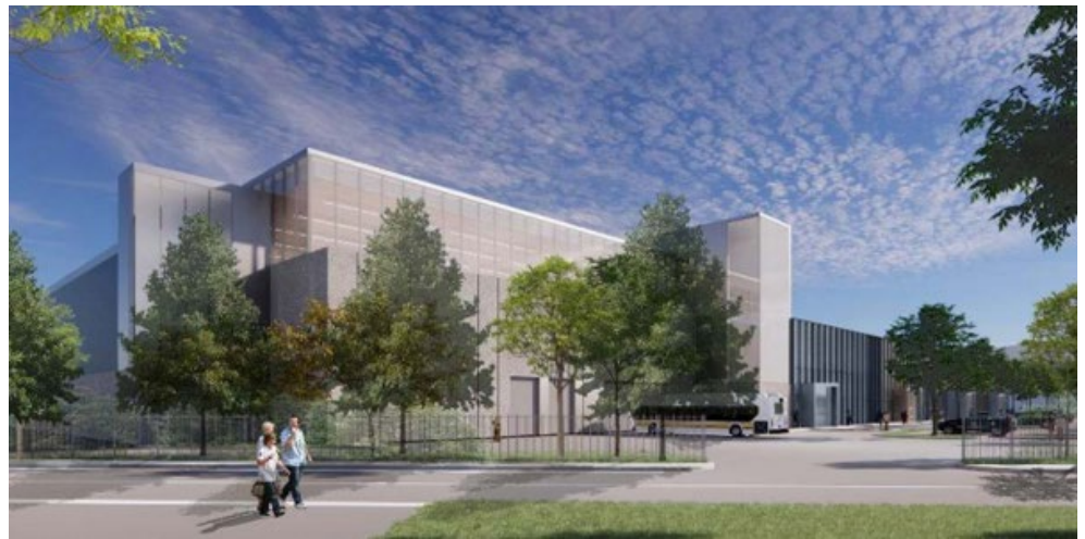
A model of the new bus facility the Massachusetts Bay Transportation Authority is building in Quincy, which will accommodate 120 battery-electric buses. Construction is set to finish in 2024, but the MBTA is planning to acquire the BEBs in winter 2022. | Massachusetts Bay Transportation Authority
