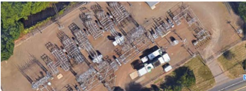
Eversource Energy wants to replace a self-contained, fluid-filled cable system with a solid dielectric cable system at a substation in Branford, Conn. | Eversource Energy
