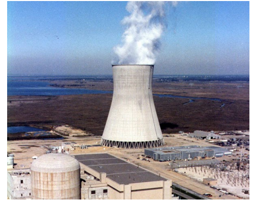
Hope Creek Nuclear Generating Station is one of two PSEG nuclear plants receiving ZEC payments from New Jersey. | NRC
