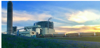
Brazos Electric has long-term PPAs for Sandy Creek's coal-fired generation. | NAES
