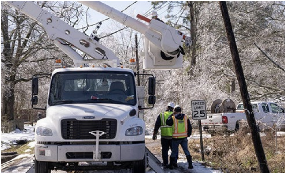
Entergy winter storm restoration last week | Entergy
