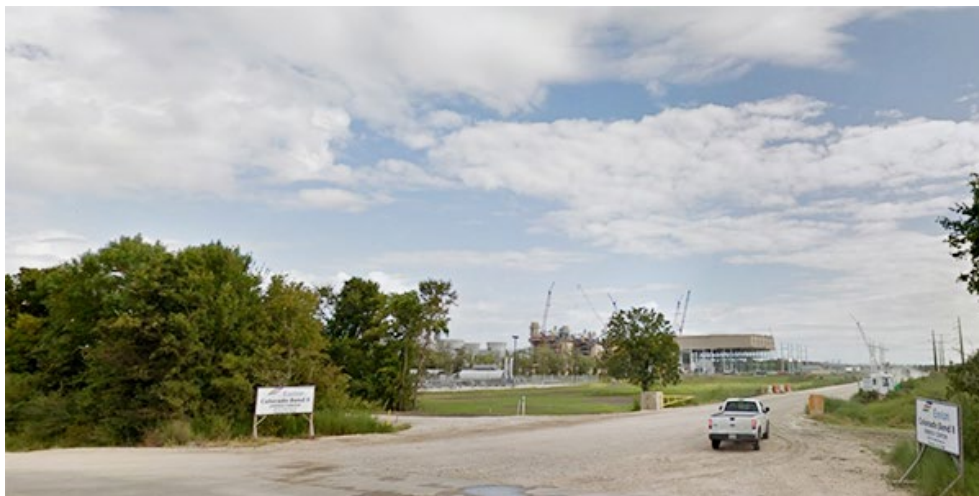
Exelon said it faces up to $950 million in pre-tax losses after three of its natural gas generators in Texas, including the Colorado Bend plant (pictured), were unable to operate during last week’s arctic freeze. | Google
