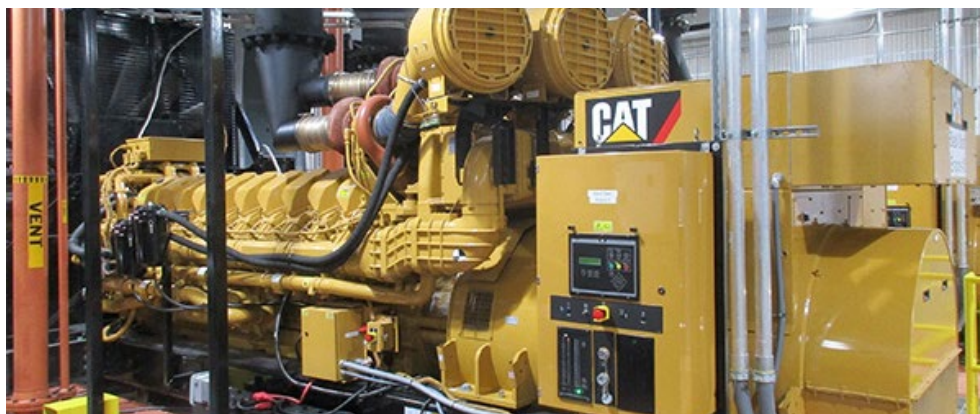
A new black start diesel engine was installed in the Carroll County Energy Center in Ohio in 2019 with the ability to provide 15.6 MW of energy in a 24-hour period. | Burns & McDonnell
