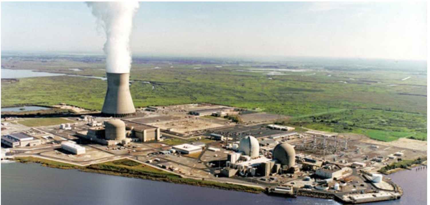
The Hope Creek and Salem nuclear units on Artificial Island in southern New Jersey | BHI Energy
