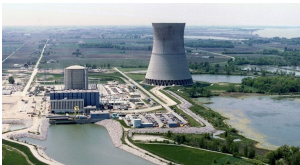
The Davis-Besse nuclear plant in northern Ohio | FirstEnergy
