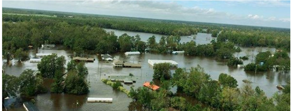
Environmental organizations in North Carolina are hoping the state will enter RGGI to help combat the effects of climate change along the state’s coastline, like the flooding seen here in 2018 from Hurricane Florence. | The Office of Connecticut Gov. Dannel Malloy
