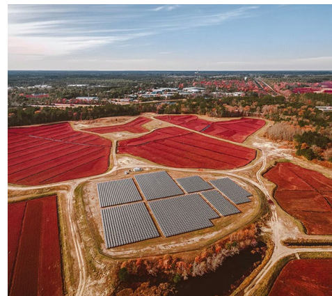
Creative project siting, like this solar farm in a cranberry bog, along with compromise between developers and communities will be critical to building out the clean generation states need to meet climate objectives. | Nexamp
