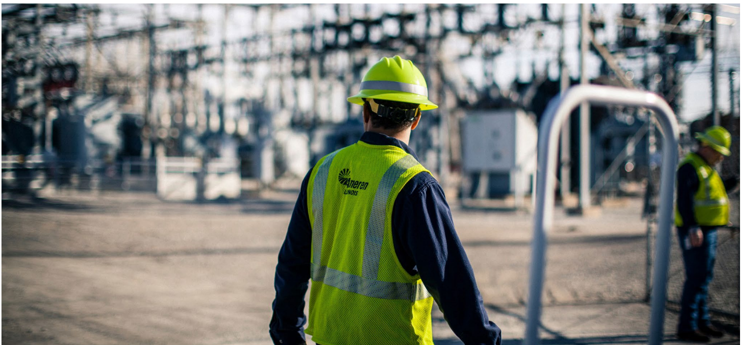
Ameren employee at a substation upgrade in 2021 | Ameren Illinois
