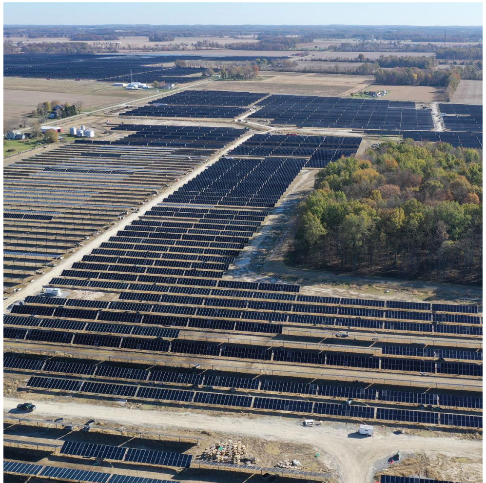
The Hillcrest Solar Project employed as many as 900 people during the peak of its construction over the last year – a timely economic stimulus to southwestern Ohio. | Innergex Renewables Development USA
