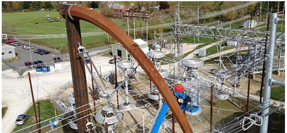
AEP transmission construction | AEP
