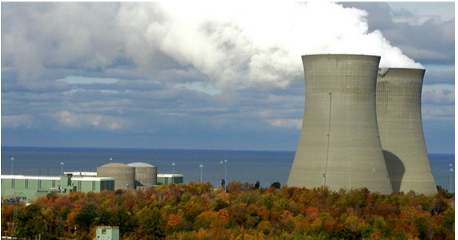
The Perry nuclear plant in Ohio | Nuclear Regulatory Commission
