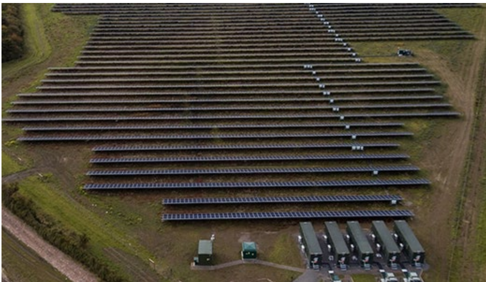
A solar farm in the U.K. co-located with energy storage | National Grid
