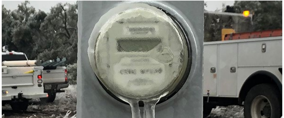
A frozen meter during the February winter storm in Texas | Kerrville Public Utilities Board
