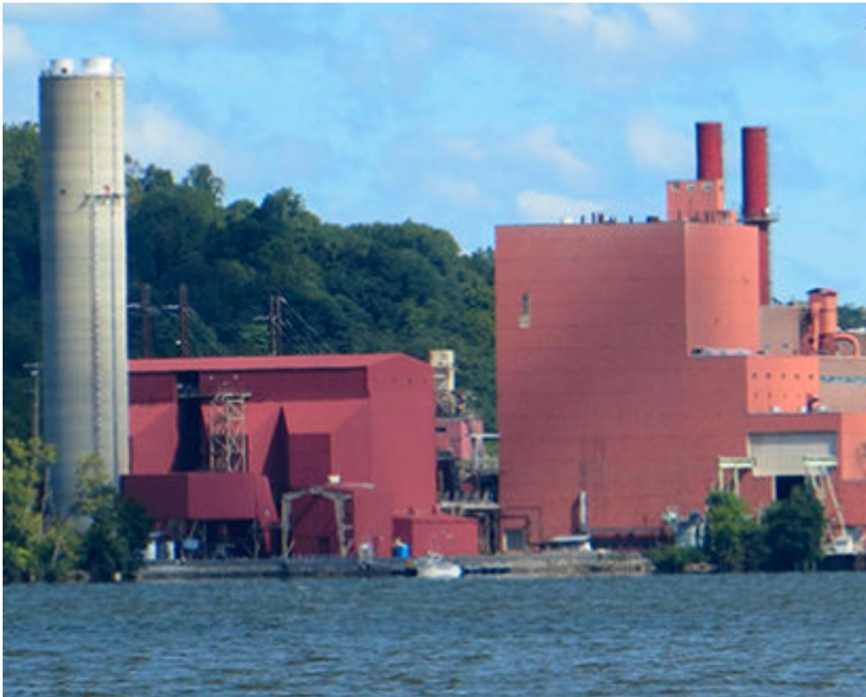
Danskammer Energy is applying to repower the 532-MW Danskammer power plant in the town of Newburgh, Orange County. | Riverkeeper
