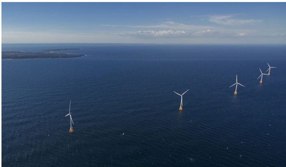
The Block Island Wind Farm, off Rhode Island | Ørsted
