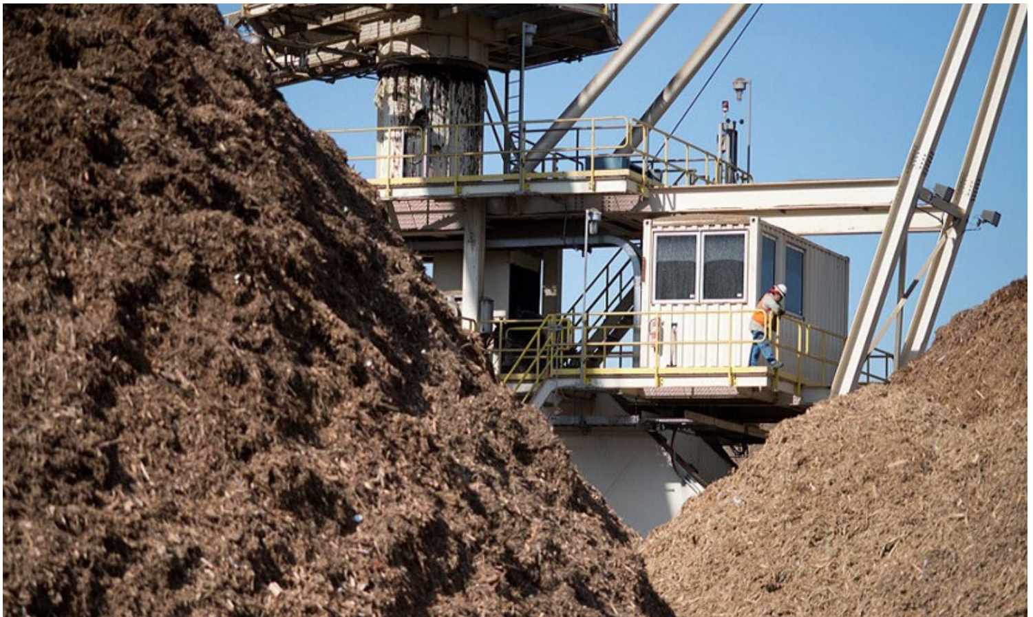
Woody biomass fuels the 44-MW Mt. Poso Cogeneration facility in Bakersfield, Calif. | DTE Energy
