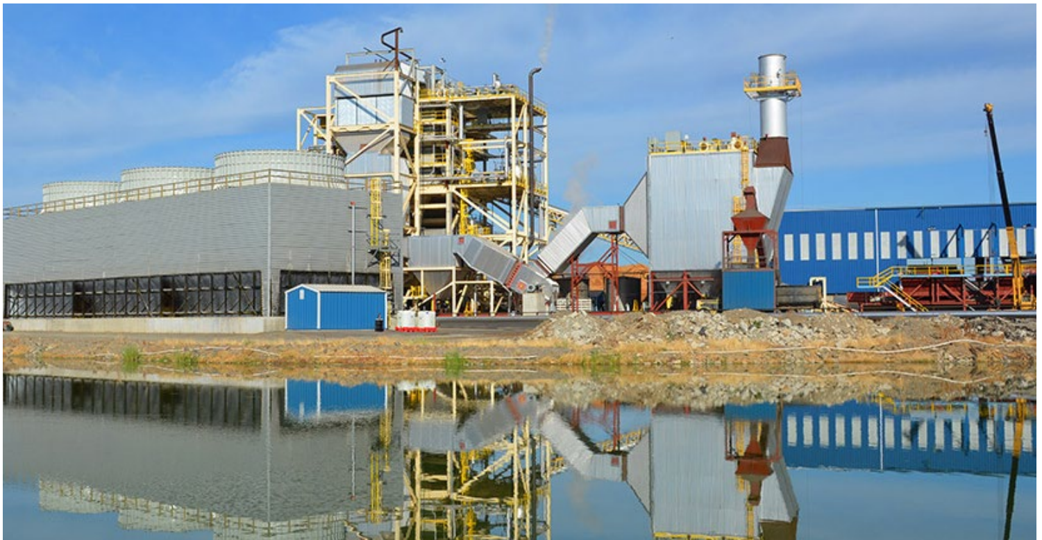
Sierra Pacific Industries operates five cogeneration facilities in California that use woody biomass from forest thinning and sawmill operations, including this plant in Shasta County. | Sierra Pacific Industries
