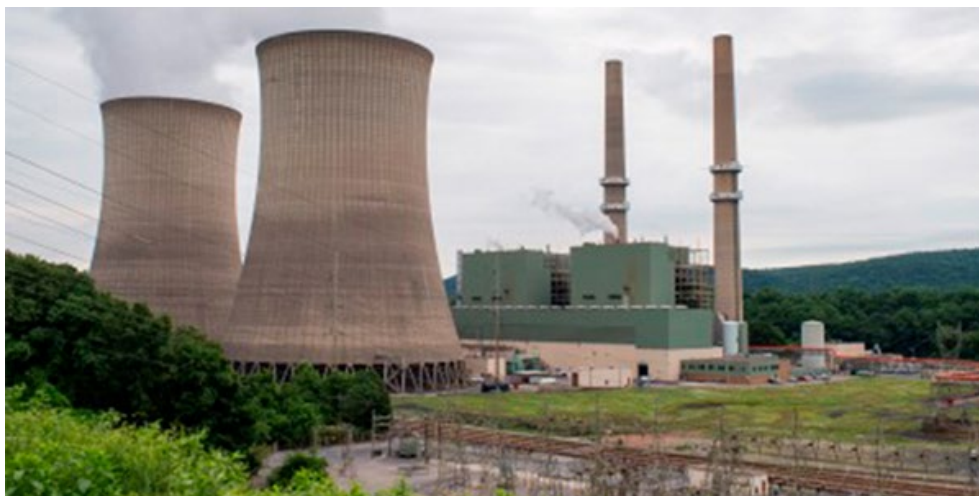
Martins Creek Power Plant in Northampton County, Pa. | Talen Energy
