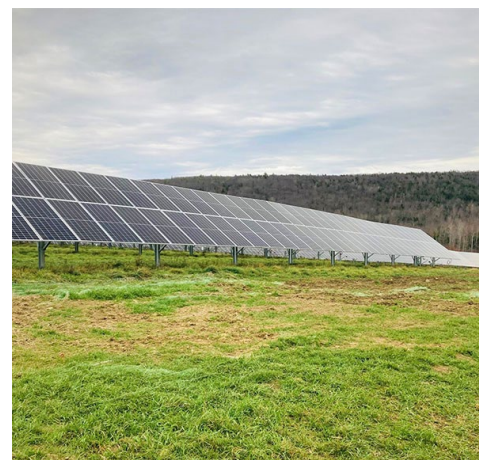
Maine regulators are investigating difficulties that planned solar arrays like this 4-MW project in central Maine are having achieving interconnection with the grid. | Revision Solar
