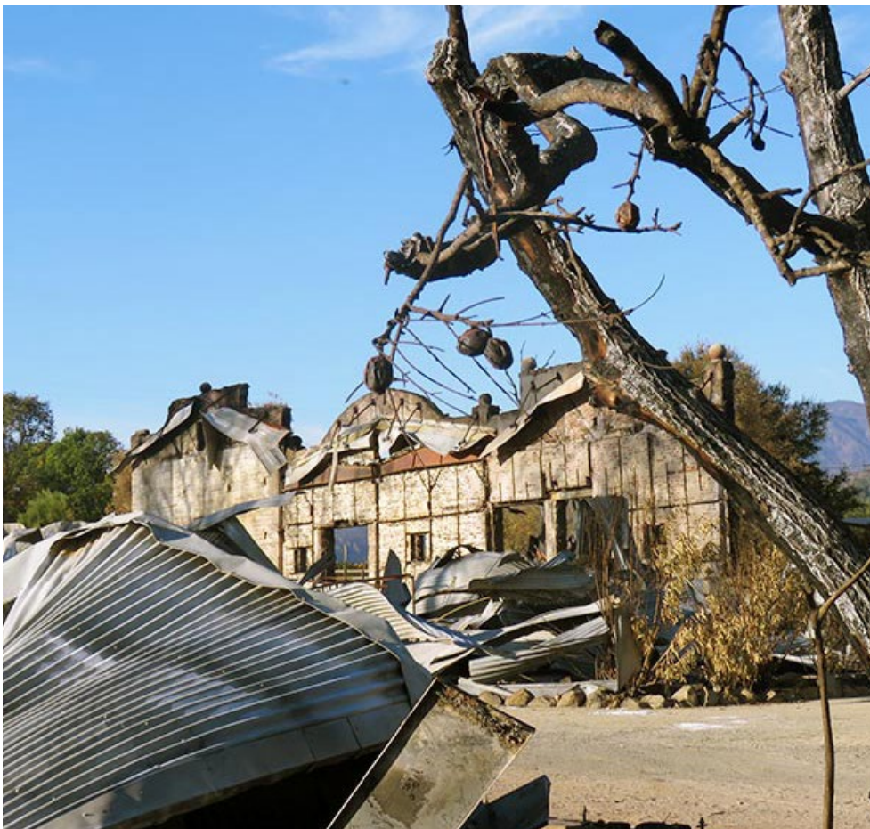
A winery from the 1800s was among the structures destroyed by the Kincade Fire. | © RTO Insider
