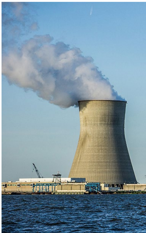
Hope Creek Nuclear Generating Station in New Jersey | Peretzp, CC BY-SA 3.0, via Wikimedia
