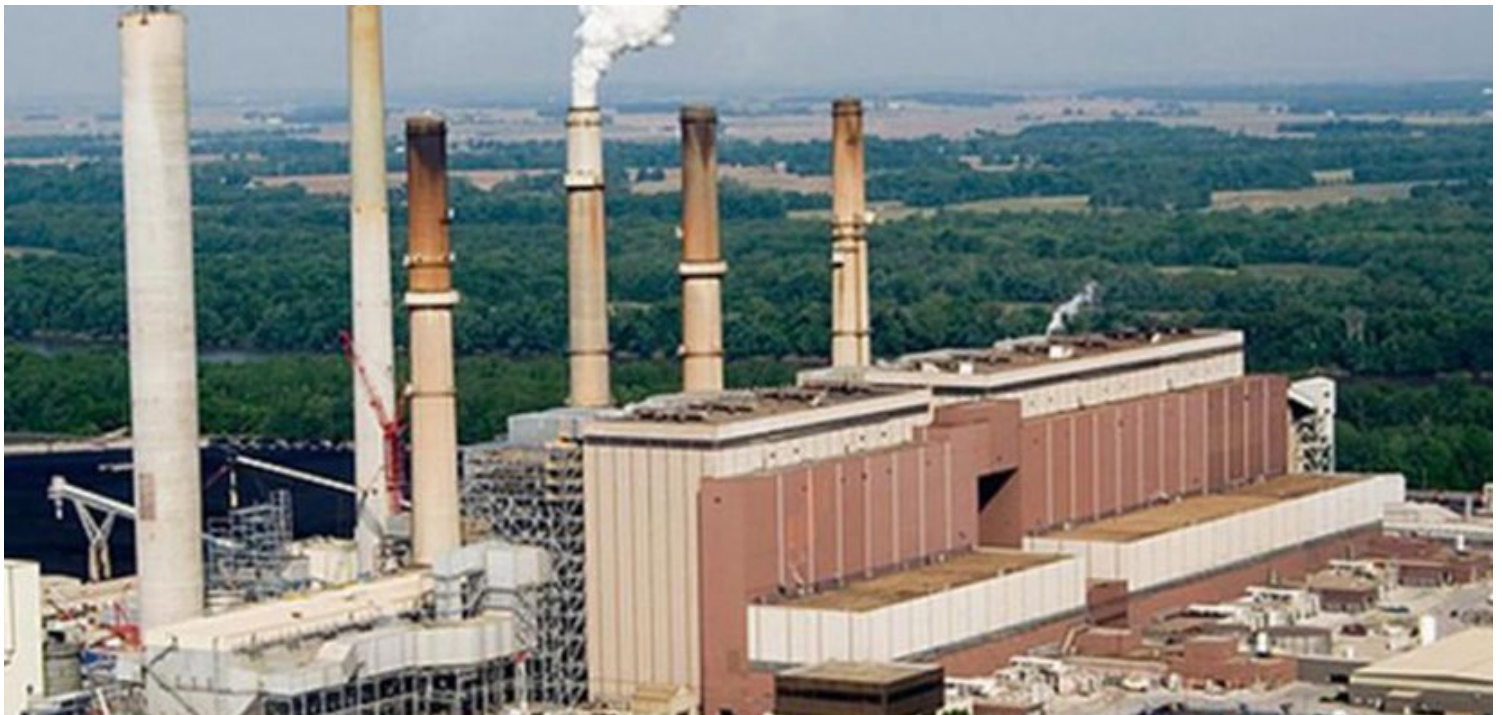
Gibson coal station | Duke Energy Indiana
