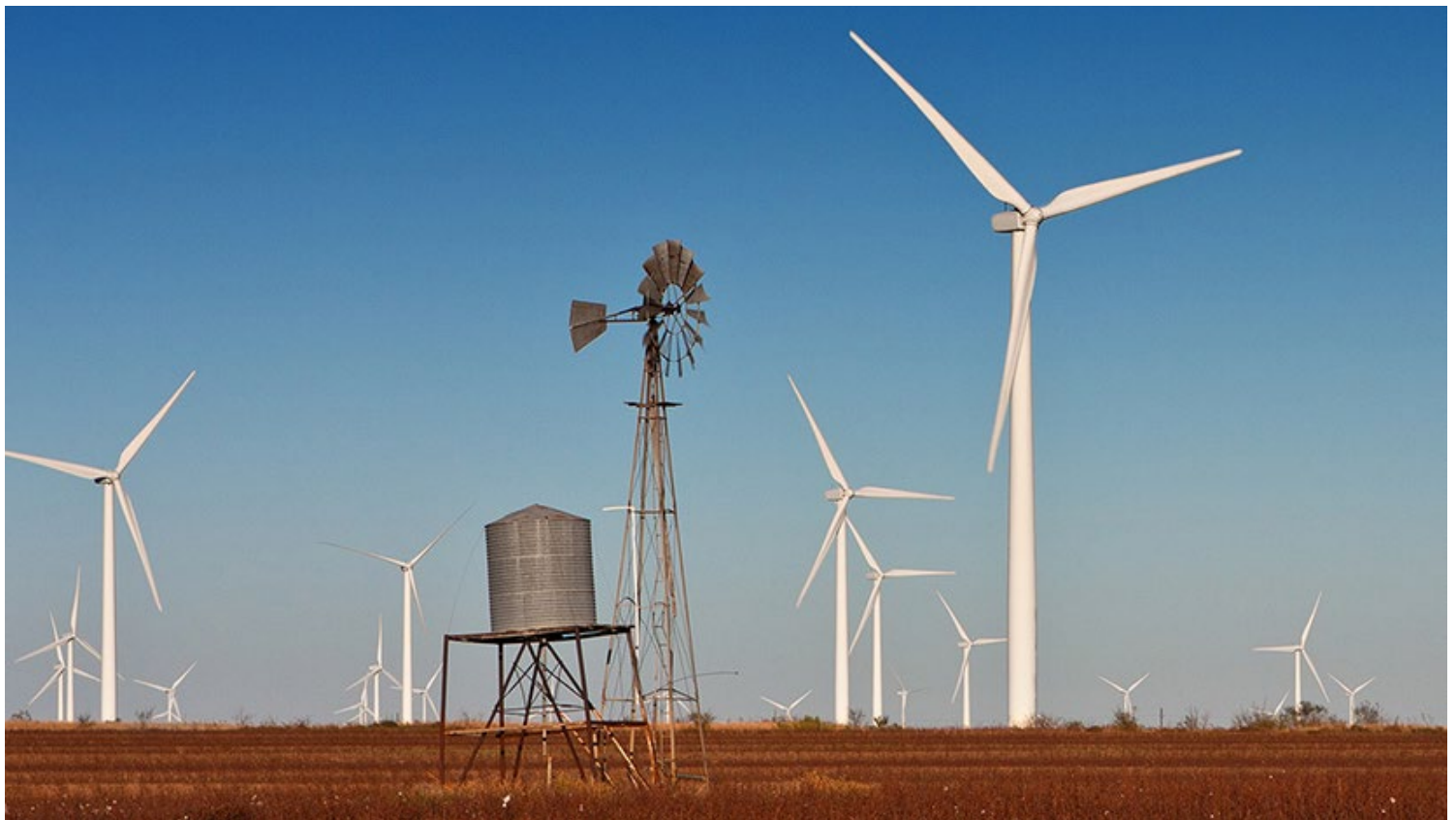
AEP has energized the first of its three North Central Energy Facilities wind farms. | Shutterstock
