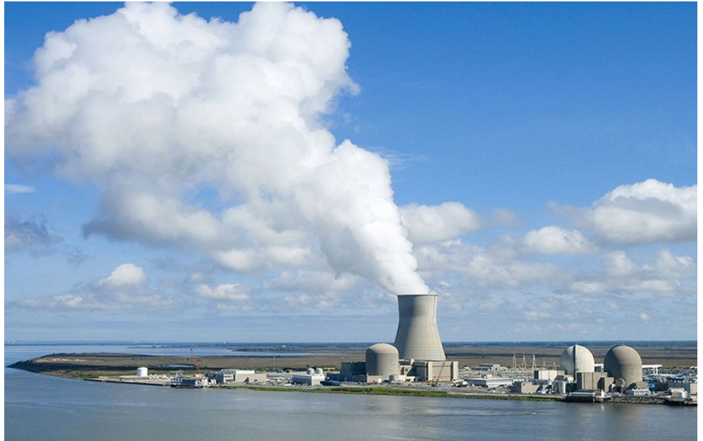
Hope Creek Nuclear Generating Station in New Jersey | Public Service Enterprise Group
