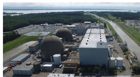
Dominion’s Surry Power Station has a capacity of 1,676 MW. | Dominion Energy
