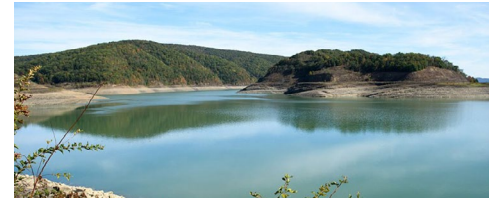
The Bath County Pumped Storage Station in Virginia's Allegheny Mountains is one of the generating plants Dominion Energy seeks to withdraw from the May 19 PJM capacity auction. | Dominion Energy
