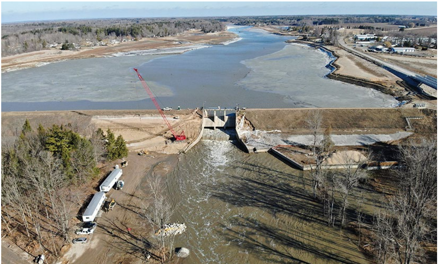
Edenville Dam following the breach | Michigan Department of Environment, Great Lakes, and Energy
