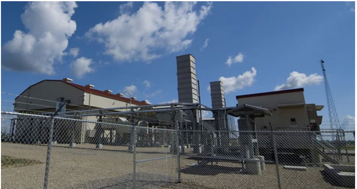
Weymouth Compressor Station | Enbridge
