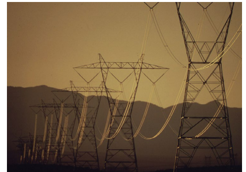
Nevada Senate Bill 448 seeks to boost the state’s transmission network and potentially place it under the oversight of an RTO. | Environmental Protection Agency
