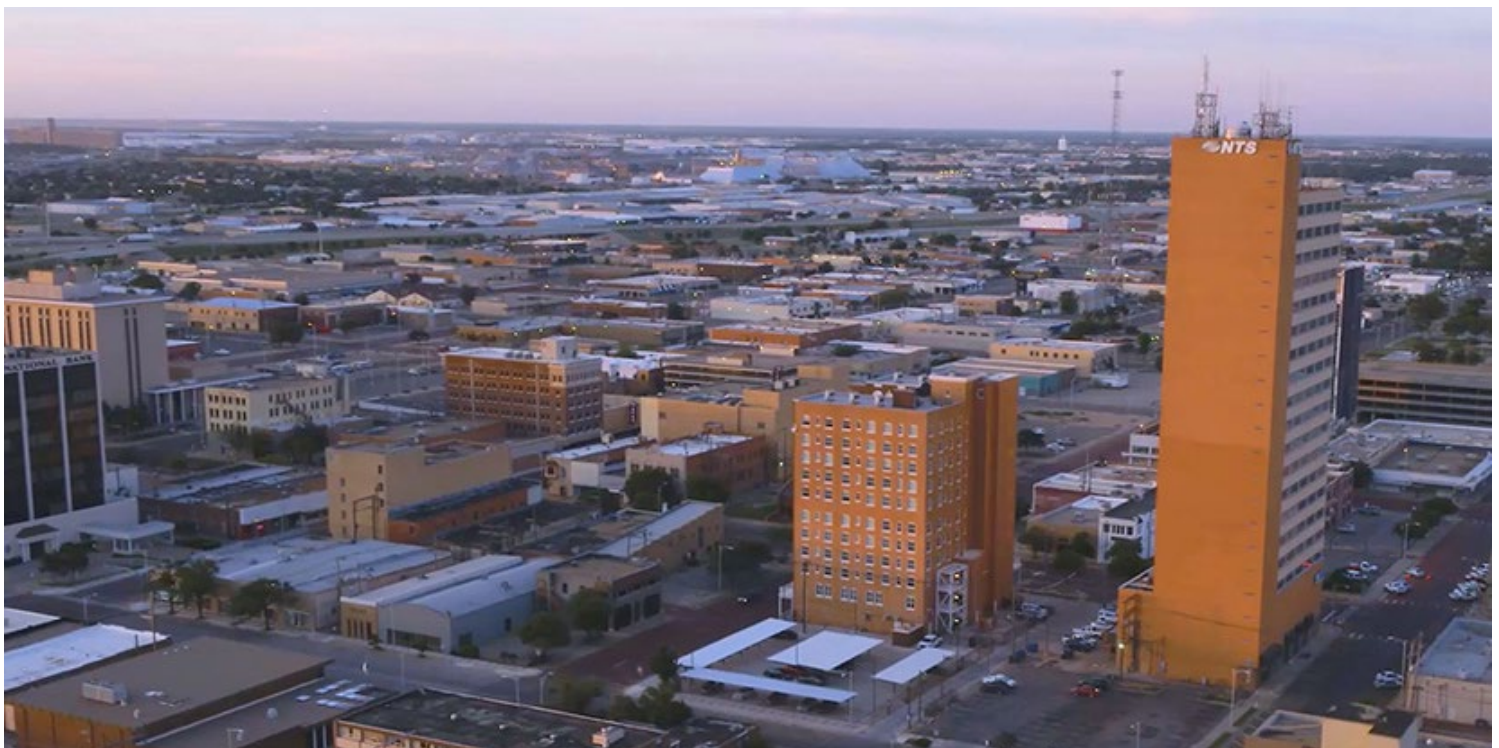
Most of Lubbock's load is now part of the ERCOT system. | City of Lubbock
