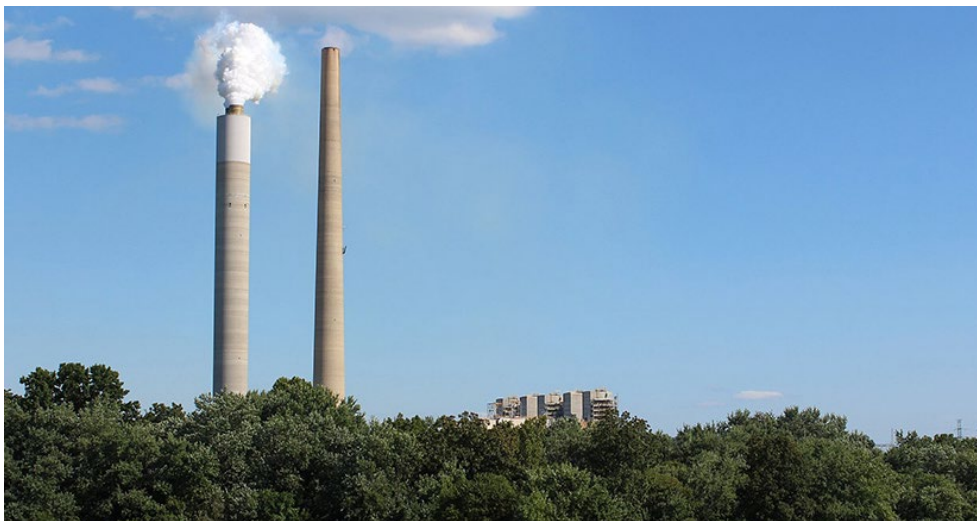
American Electric Power is part owner of the Kyger Creek Generating Station in Ohio, which received a subsidy from a controversial 2019 state law. | FunksBrother, CC BY-SA 4.0, via Wikimedia Commons
