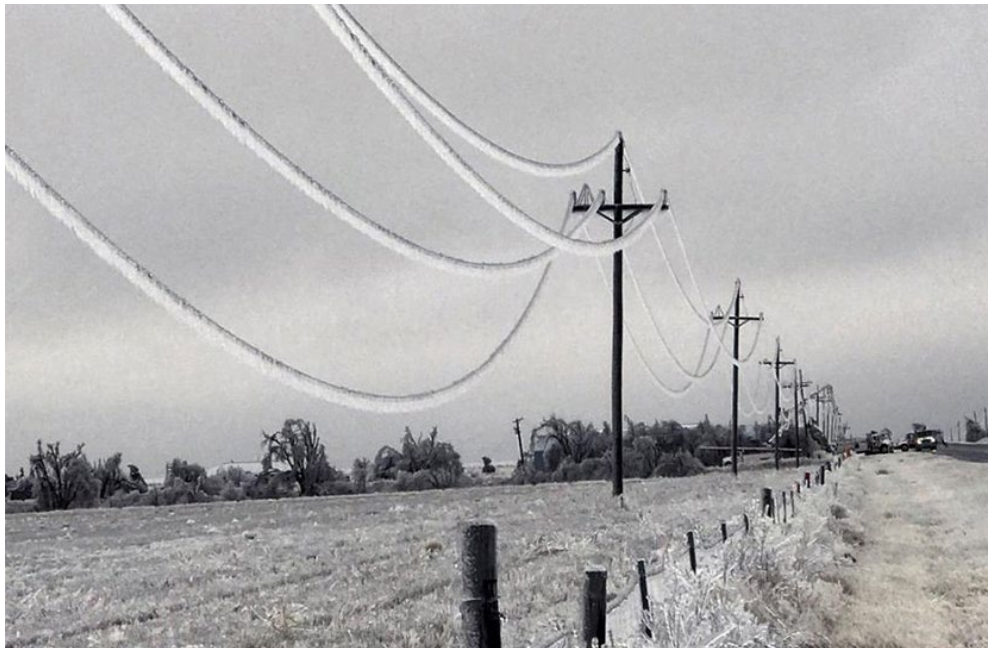
Ice-covered Texas transmission lines | Xcel Energy
