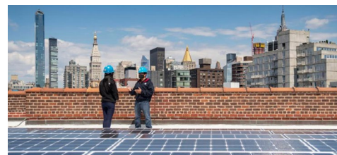
Con Edison workers at a solar installation at Peter Cooper Village in Manhattan | Con Edison
