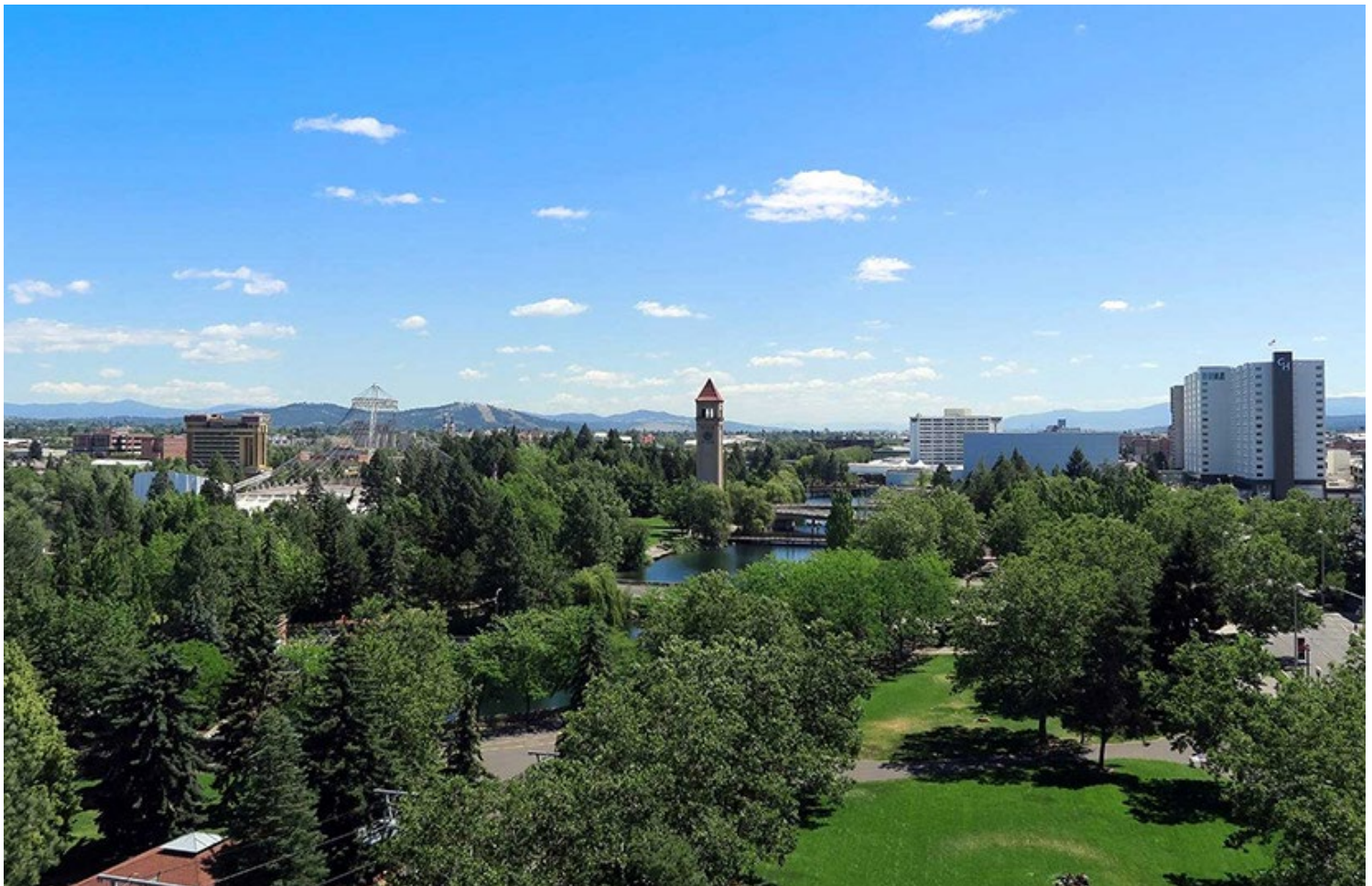
Avista implemented rolling blackouts in Spokane, Wash., on June 28 in the face of record heat. | City of Spokane
