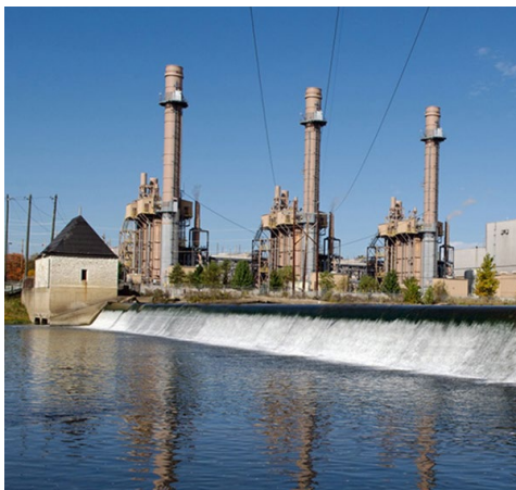
Noblesville Station in Hamilton County, Indiana | Duke Energy
