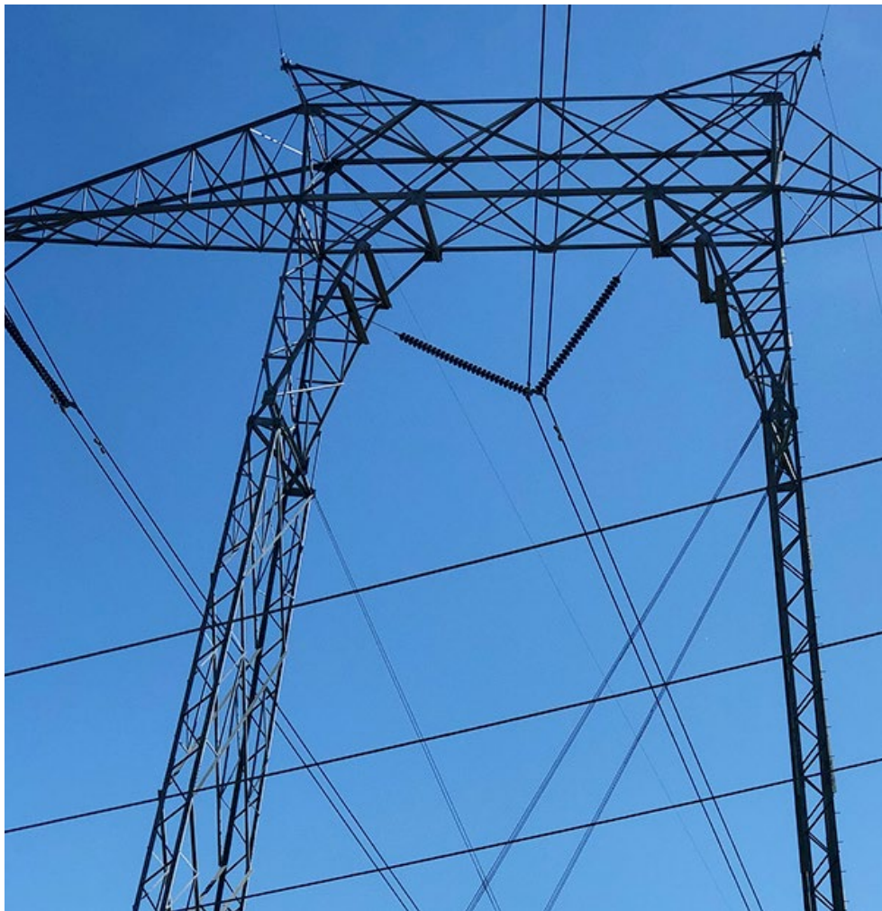
A main north-south transmission line runs through Sutter County, Calif. | © RTO Insider LLC
