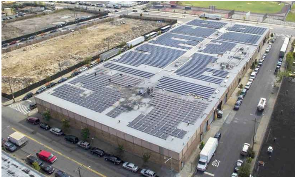
Liberty Distributors in Brooklyn expanded its solar installation to 626 kW in 2018 to create a new source of revenue. | 174 Power Global
