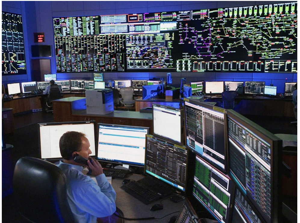
PJM control room | PJM
