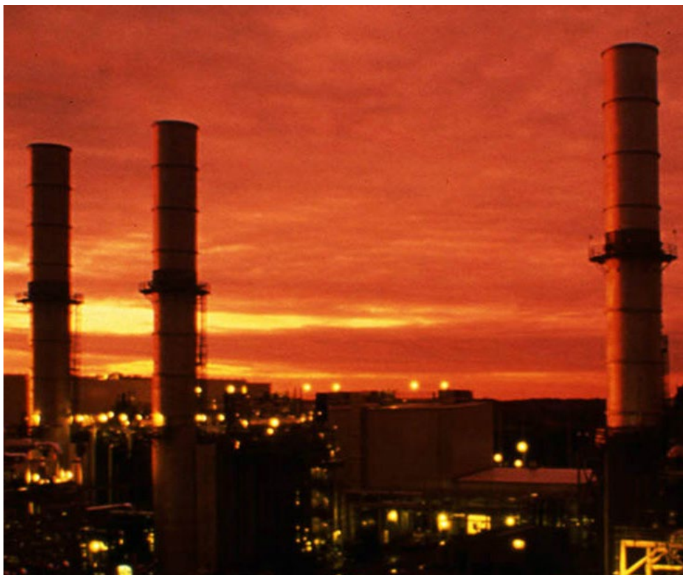
Originally constructed as a 665-MW combined cycle plant (pictured), the Doswell gas-fired generator in Virginia was expanded by LS Power with the addition of two 170-MW peaking plants. | Fluor
