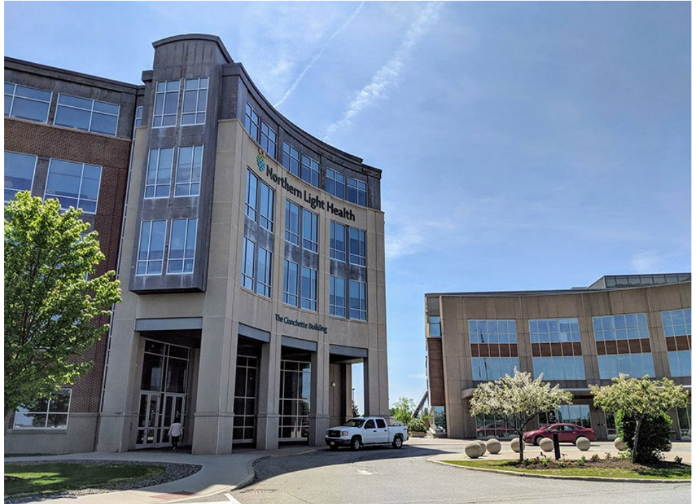
Northern Light Health, one of the largest hospitals in Maine, could qualify for a new energy storage pilot program that will target critical facilities that are sophisticated energy consumers. | Northern Light Health
