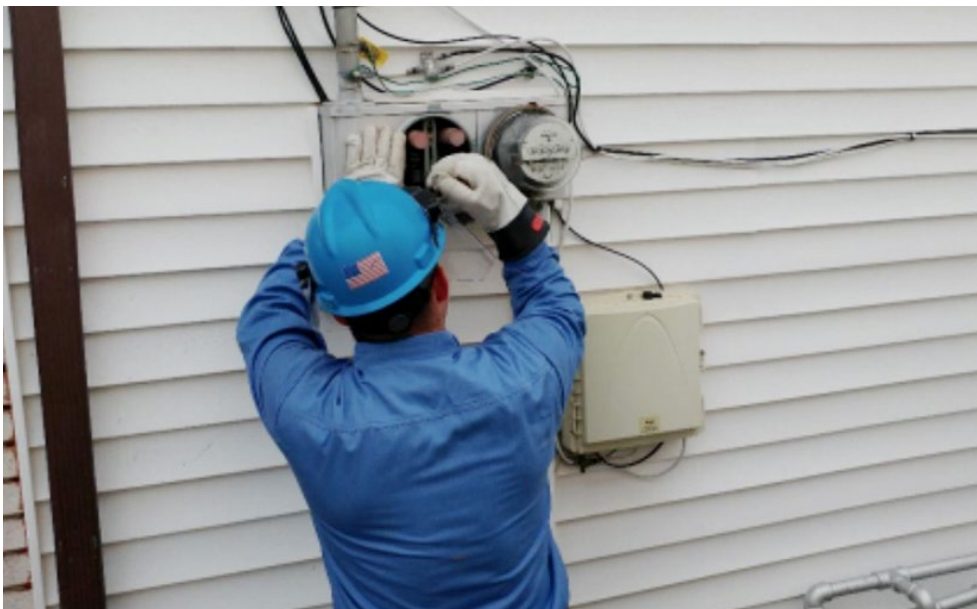
A Con Edison worker connects an adapter that uses the residential electric meter socket as a point of interconnection for solar power. | Con Edison
