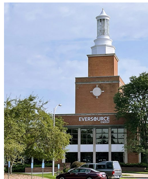
Eversource Energy's Berlin, Conn., campus | © RTO Insider LLC
