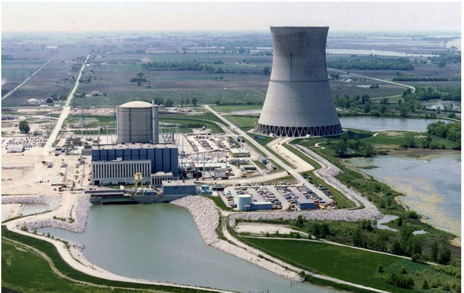
Davis-Besse nuclear plant in northern Ohio | NRC
