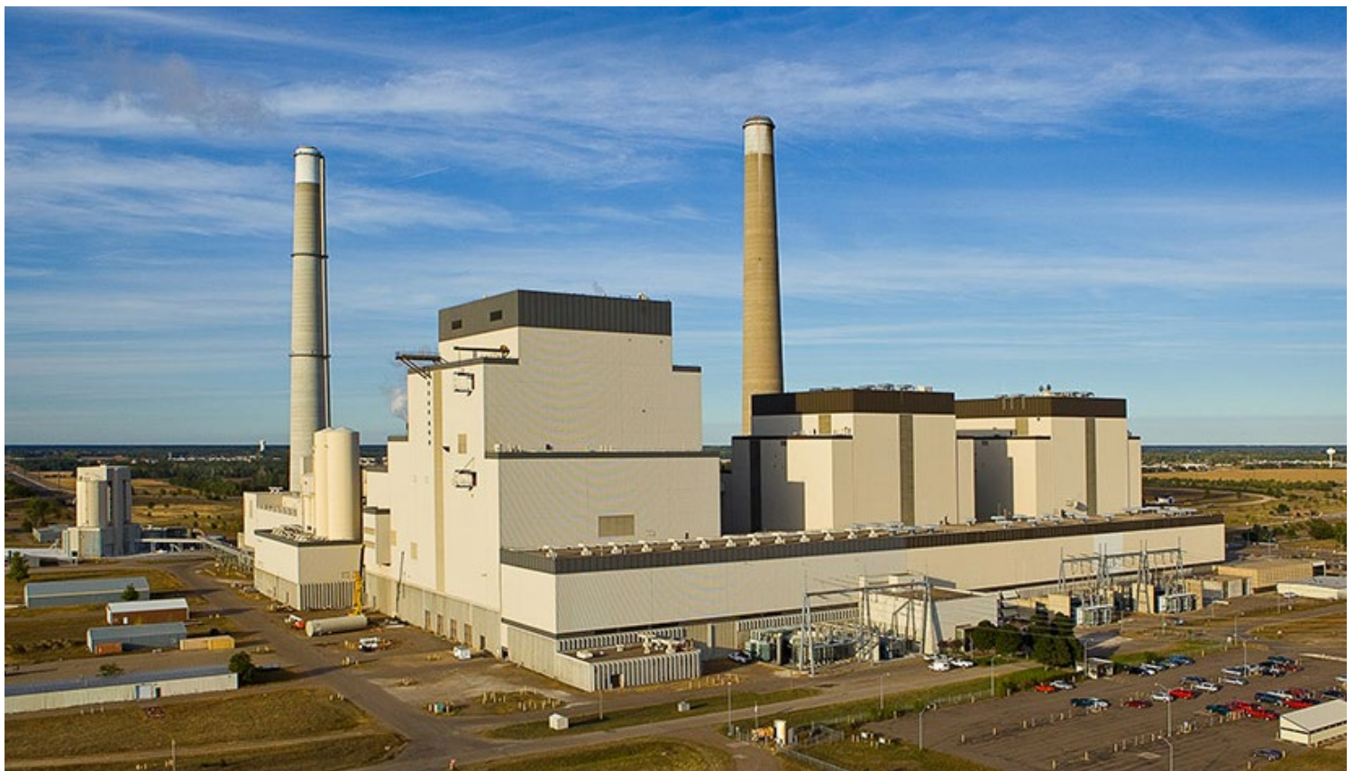
Xcel Energy's Sherco power plant in Becker, Minn. | Xcel Energy
