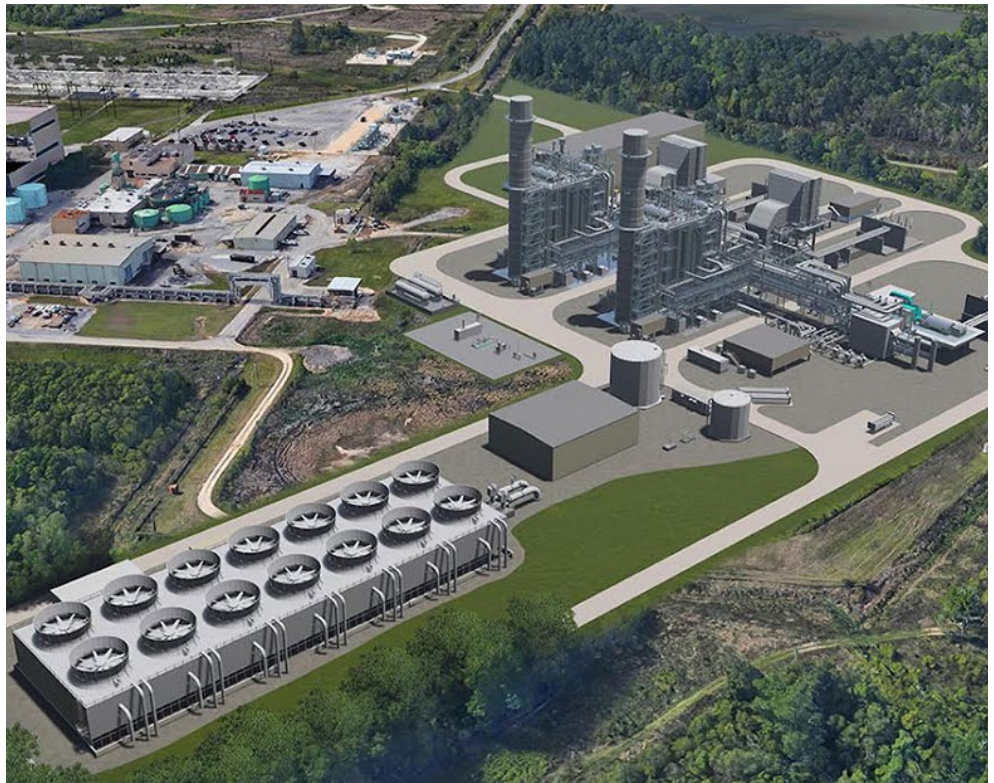
Entergy hydrogen plant | Entergy
