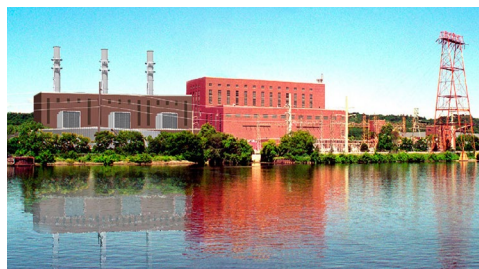
PSEG's Bethlehem Energy Center, an 817-MW combined cycle plant in New York | PSEG
