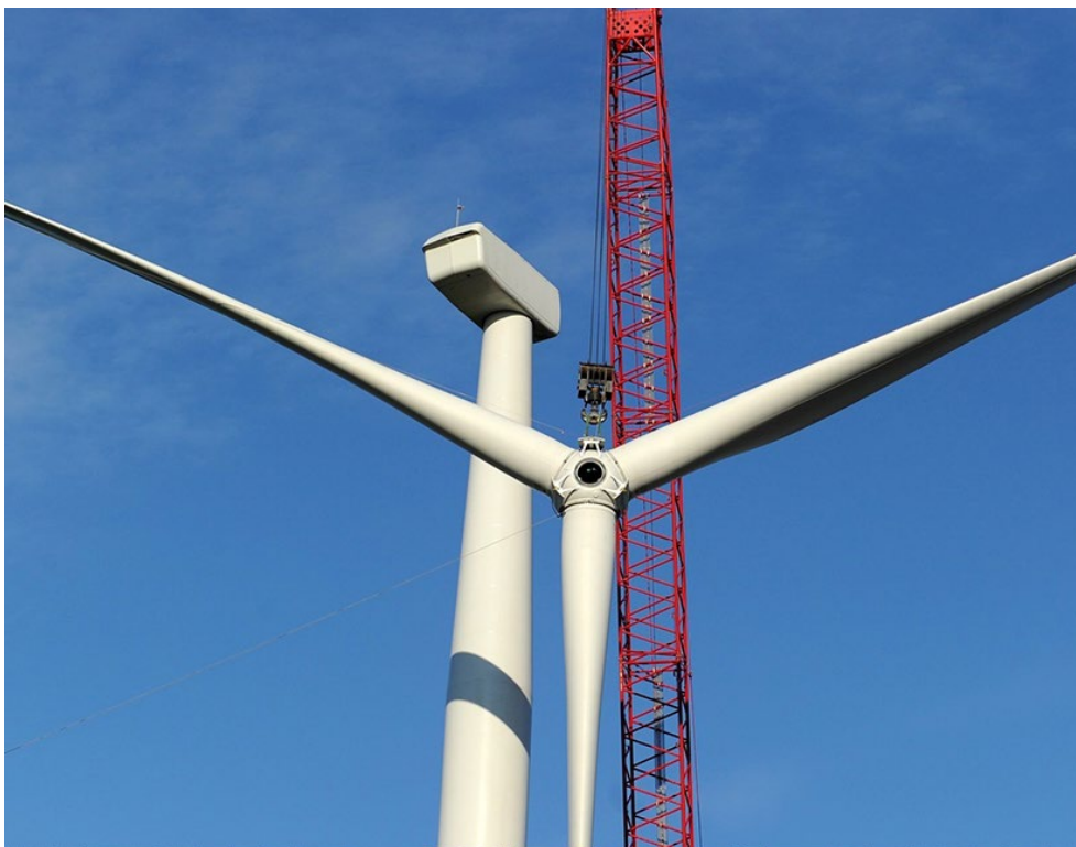
Construction of DTE Energy's Meridian Wind Park | DTE Energy
