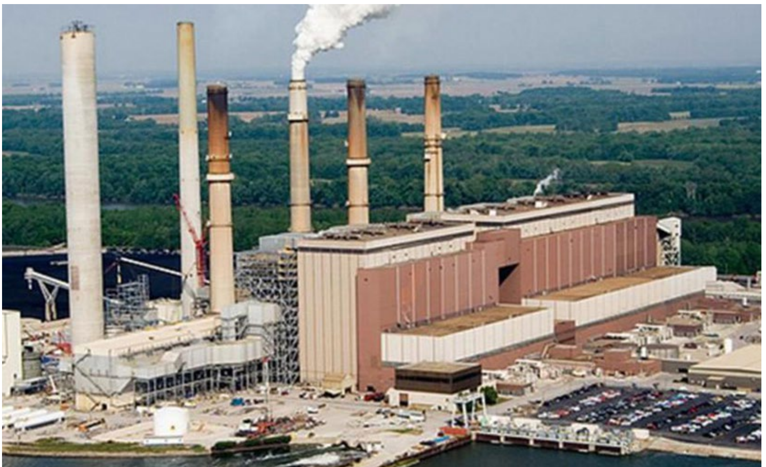
Gibson coal station | Duke Energy Indiana
