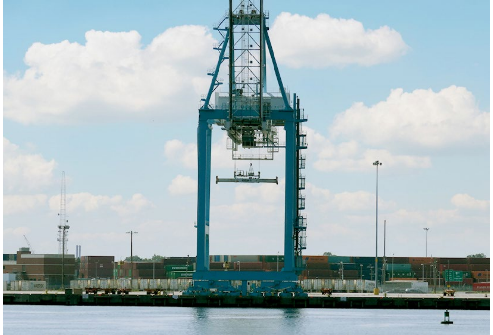
Dominion Energy will use the Portsmouth Marine Terminal in Virginia, seen here Aug. 24 during a port tour organized by the utility for the International Partnering Forum, as a staging and pre-assembly area for foundations and turbines. | © RTO Insider LLC
