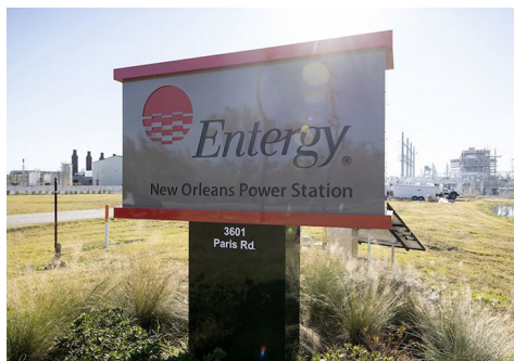
Entergy's New Orleans Power station was brought online in May 2020. | Entergy
