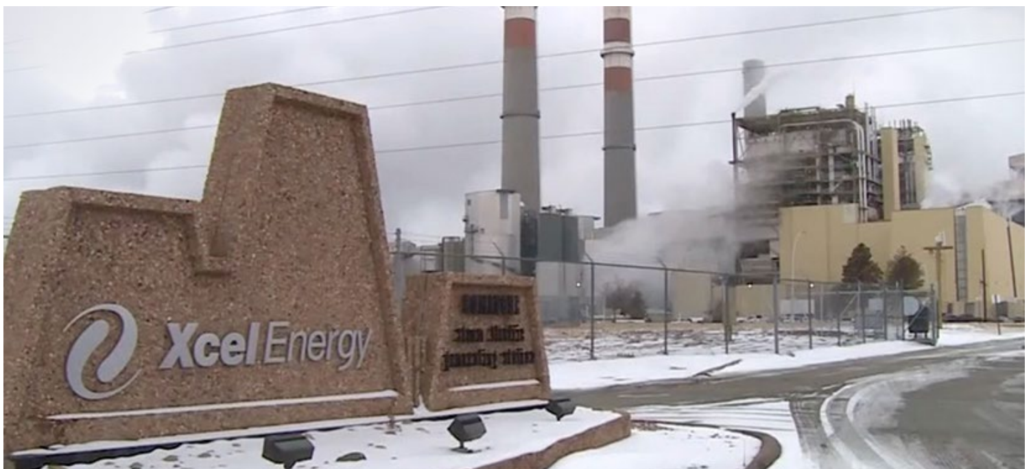
Xcel Energy's Comanche 3 coal plant | KRDO
