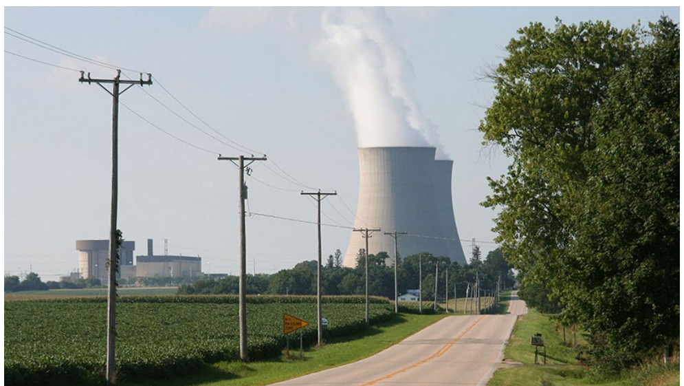
Unit 1 of Exelon's Byron nuclear power plant in Illinois shut down early Monday for re-fueling or for decommissioning if Illinois lawmakers failed to approve legislation providing nearly $700 million in public funding over six year for its Byron and Dresden nuclear plants that the company said cannot compete against gas turbines and subsidized renewable energy | Ben Jacobson, CC BY-2.5, via Wikimedia
