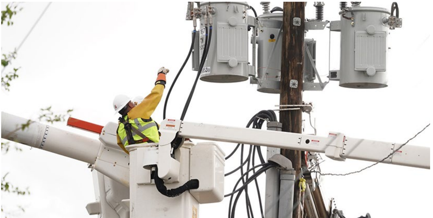
Hurricane Ida restoration | Entergy
