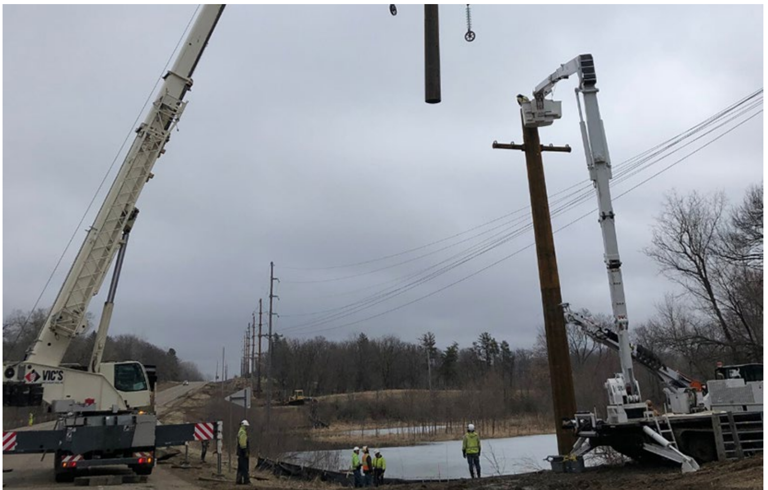
Great River Energy line construction in 2020 | GRE
