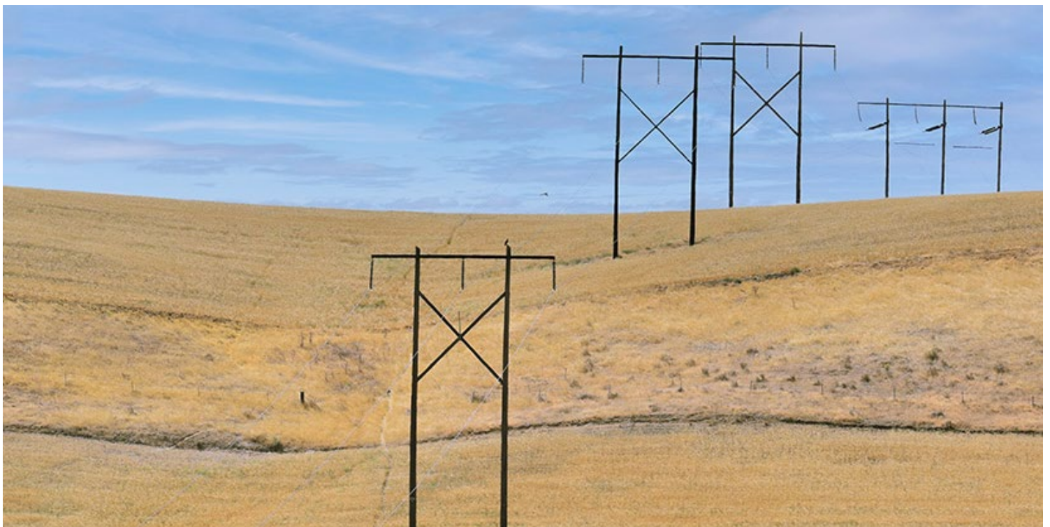
Transmission line in Umatilla County, Oregon. | © RTO Insider LLC
