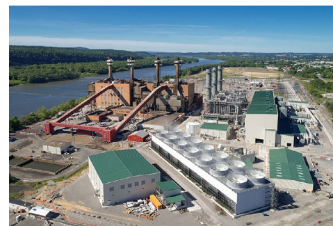
Panda Hummel Station, a 1,096.5-MW combined cycle plant on the Susquehanna River near Sunbury, Pa. | Bechtel Corp.
