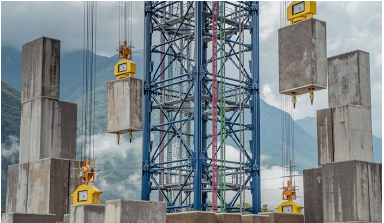
The DOE wants long-duration storage technologies — like Energy Vault’s towers that raise and lower 35-ton blocks of concrete — to hit a levelized cost of $0.05 per kWh-cycle for 10 hours or more within the next decade. | Energy Vault
