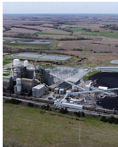
Sheldon coal generating station near Lincoln, Neb. | Nebraska Public Power District
