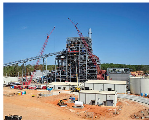
Austin Energy's Nacogdoches Power under construction | Southern Power
